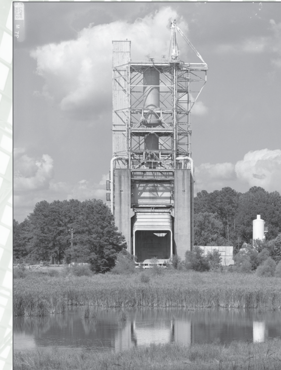
NASA Marshall Space Flight Center, F-1 Engine Static Test Stand, Huntsville vicinity, Alabama, Jet Lowe, photographer, 2009. HAER has had a long-term partnership with Marshall Space Flight Center documenting its national landmarks and other historic resources.
