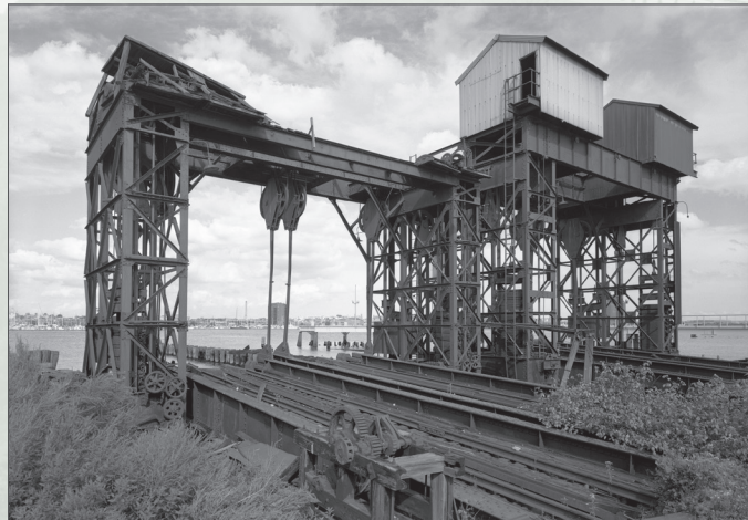
Baltimore & Ohio Railroad, Locust Point Float Bridges, Baltimore, Maryland, Jet Lowe, photographer, 2011. A vestige of railroad infrastructure, this floatbridge was once used to transfer freight cars onto rail-equipped barges called carfloats.
