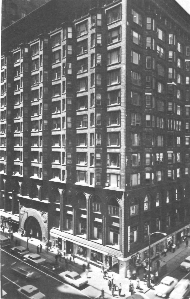
Louis Sullivan's Chicago Stock Exchange, now threatened by demolition.
