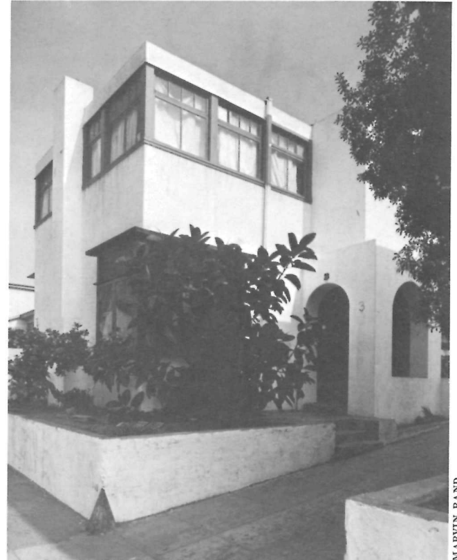
Horatio West Court, Santa Monica, Calif. Irving J. Gill, architect.
