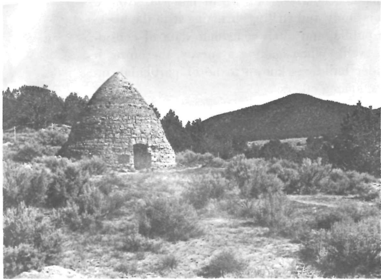
Coke Oven, Old Irontown, Utah. This early industrial remain was built in 1869 by the Union Iron Works, which had been organized the year before.
