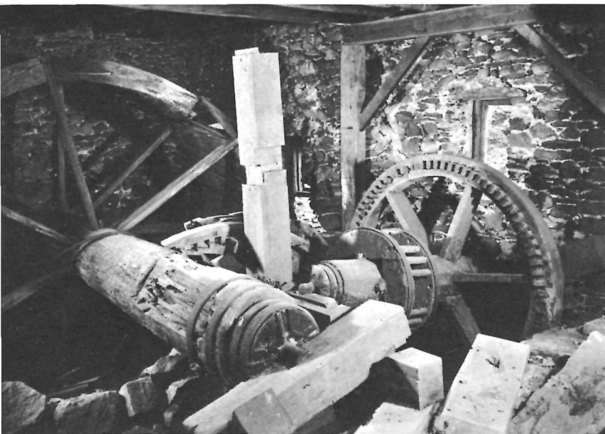
Thomas Mill, Edgemont Vicinity, Chester County, Pa. Basement, toward water wheel.
