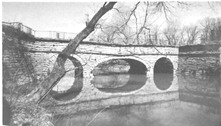
Chesapeake and Ohio Aqueduct over Catoclin Creek, Point of Rocks, Md.
