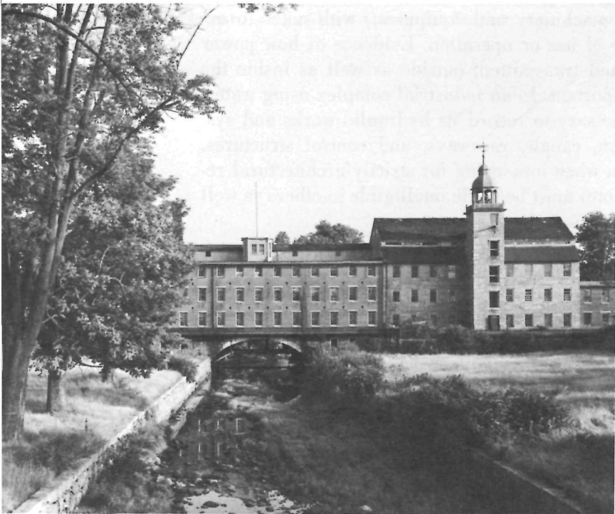
Crown and Eagle Mills, North Uxbridge, Mass. An independent cotton mill in a rural setting, consisting of portions built in 1823, 1827, and 1851. It is a prime exemplar of its kind.
