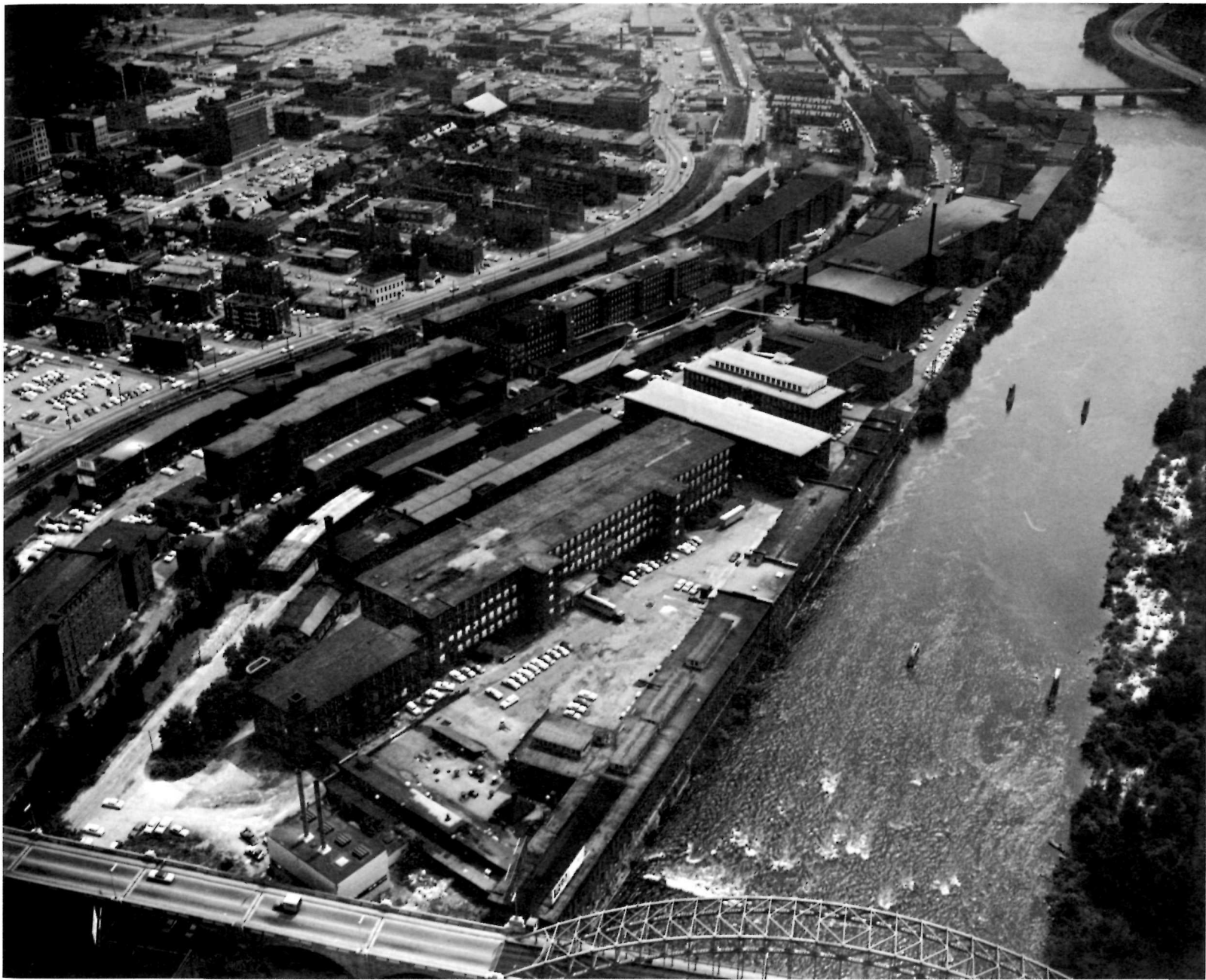
Amoskeag Mill Complex, Manchester, N.H. View from a helicopter.
