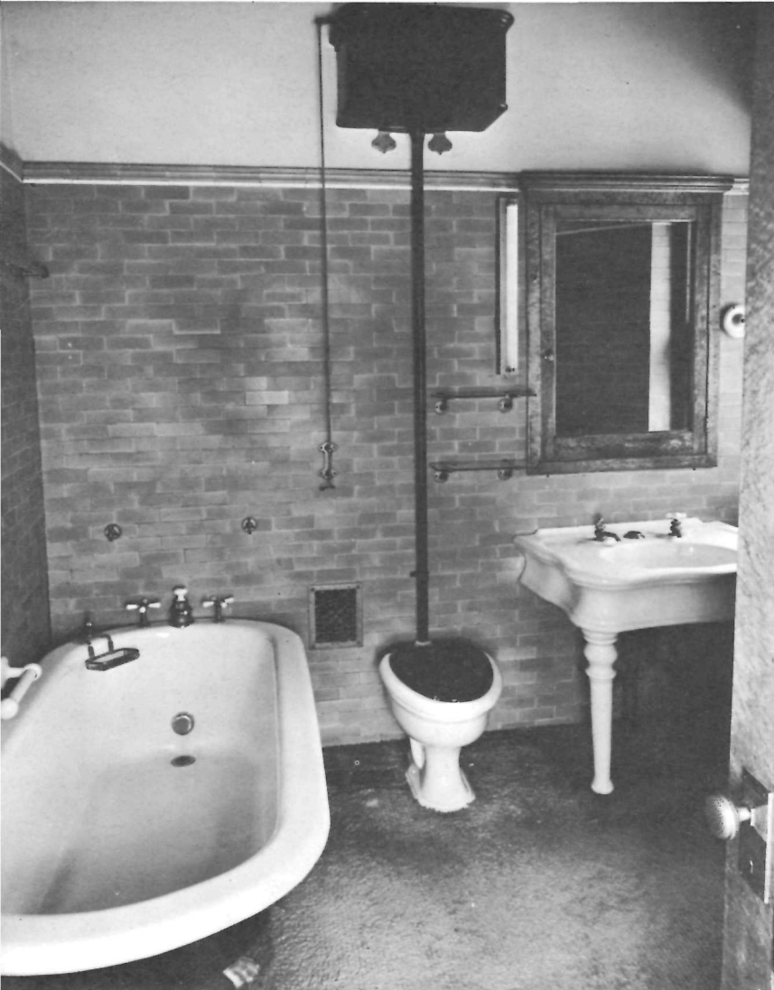
Edward E Ayer House, Chicago, Ill. Bathroom.
