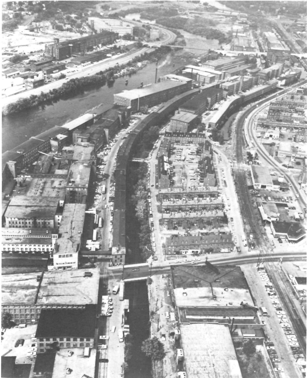
Amoskeag Mill Complex, Manchester, N.H. A low-level oblique aerial view taken from a helicopter, which shows the buildings being recorded in context with the setting.
