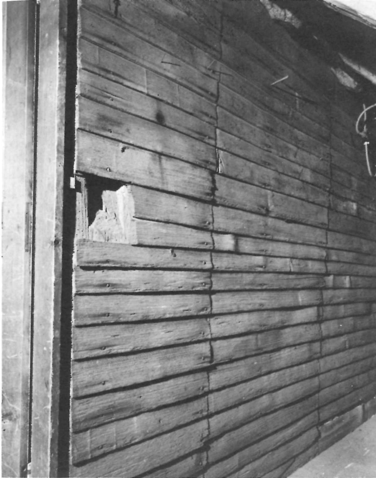
Robert Pierce House, Dorchester, Mass. Cedar clapboarding preserved in attic of lean-to. It is unusual to find remains of clapboarding as old as the 17th century.
