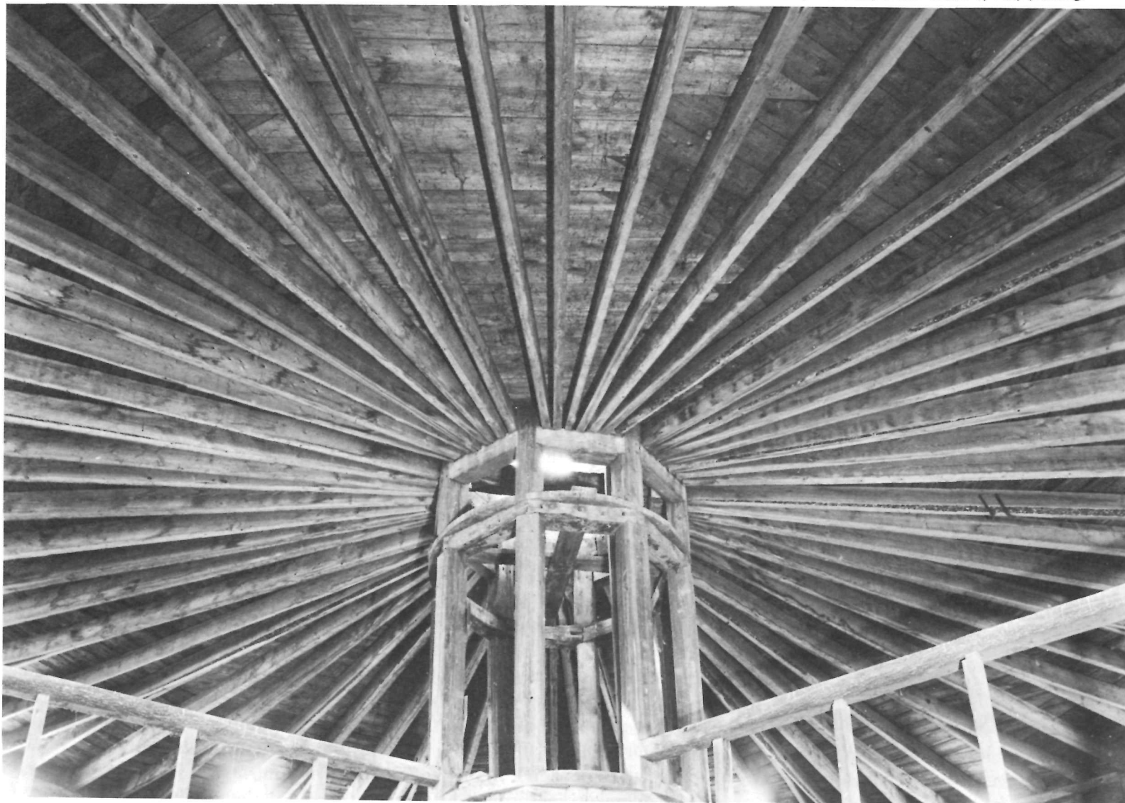
Hancock Shakers' Round Barn, Hancock, Mass. Detail of roof framing.
