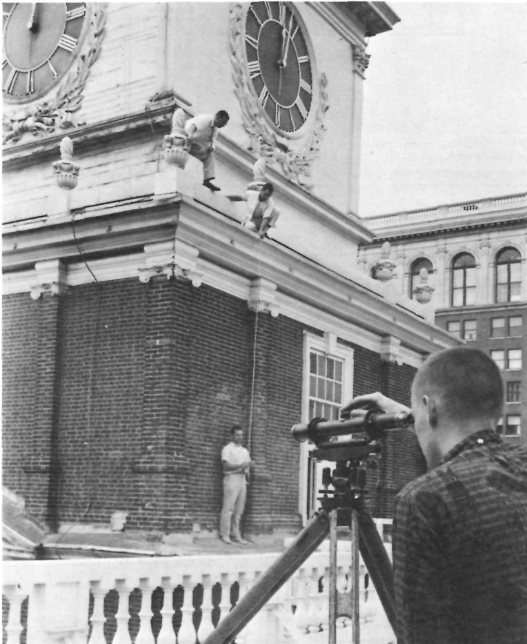
Use of a surveyor's level: HABS team at Independence Hall, Philadelphia, Pa.
