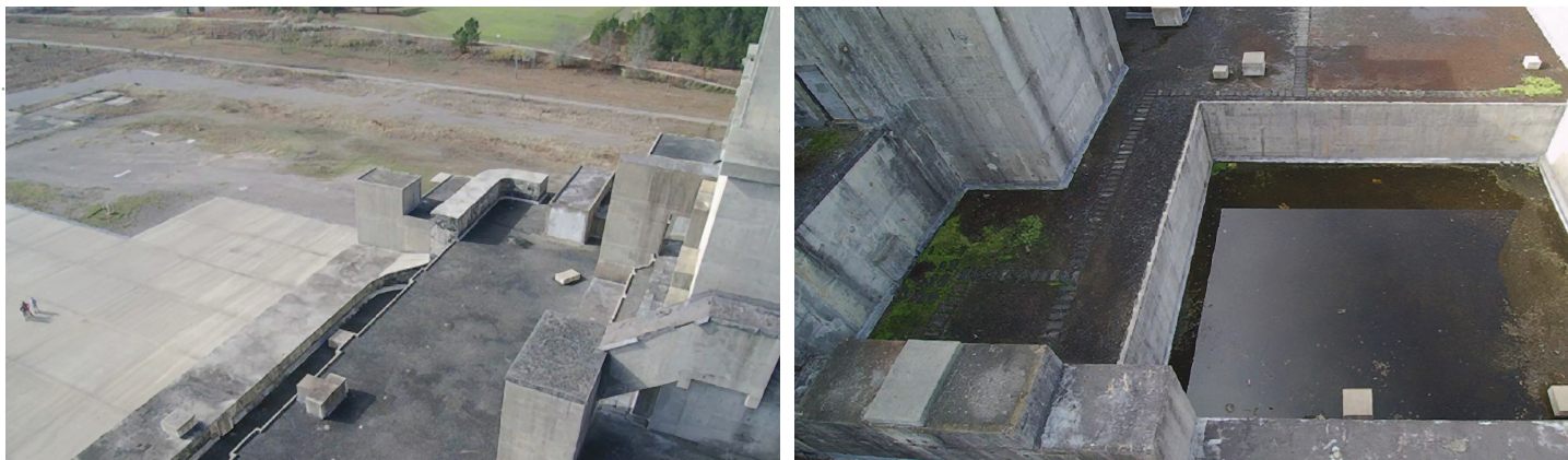
Top Left: Unmanned aerial vehicle view of SRNL operators from above an entombed reactor building at SRS; Top Right: Potentially intrusive vegetative growth on entombed nuclear reactor building recorded by unmanned aerial vehicle
