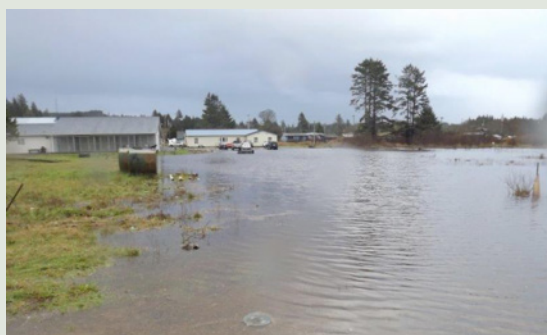
Figure 24.10: Coastal floodwaters inundated the Quinault Indian Nation's lower village of Taholah in March 2014. This event, and continuing concerns about future climate change, prompted the village to begin relocation to higher ground. Photo credit: Michael Cardwell.
