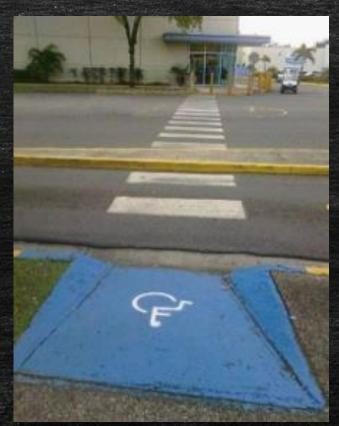
Image description: A blue curb cut with the wheelchair access sign leading to a crosswalk. The street has a curb blocking the crosswalk.
