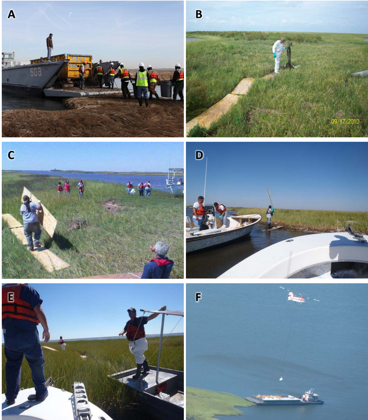
Figure 3. Examples of equipment and removal methods suitable for removal of debris items from interior of vegetated wetlands including via manual removal to shallow draft vessel (A), use of walking boards (B-E) and helicopter sling load (F). Photo credits: RPI, USFWS.
