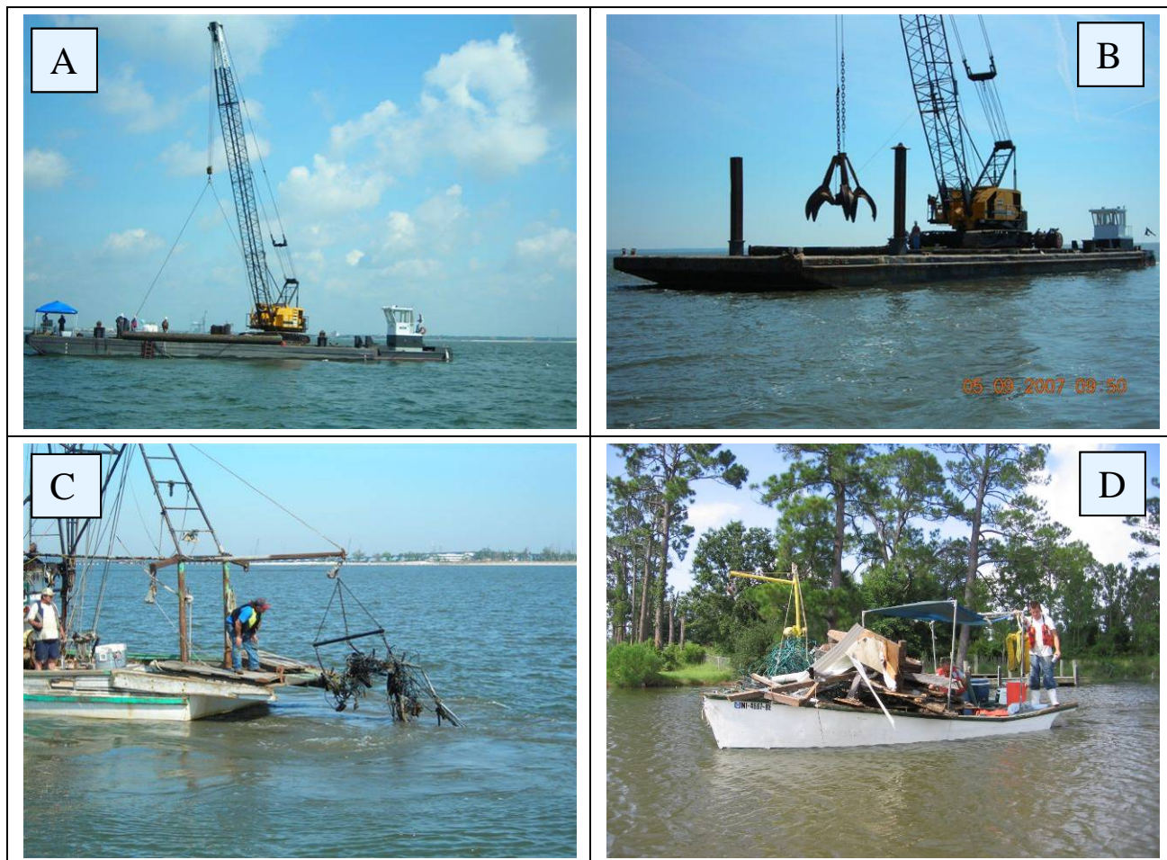
Figure 14. Marine debris removal methods. A. Crane on a barge picking up larger items. B. Large grappling device in a point-pickup removal. C. Small grappling hooks. D. Shallow-draft vessels transporting marine debris from creeks. Photograph credit: USCG and NOAA.
