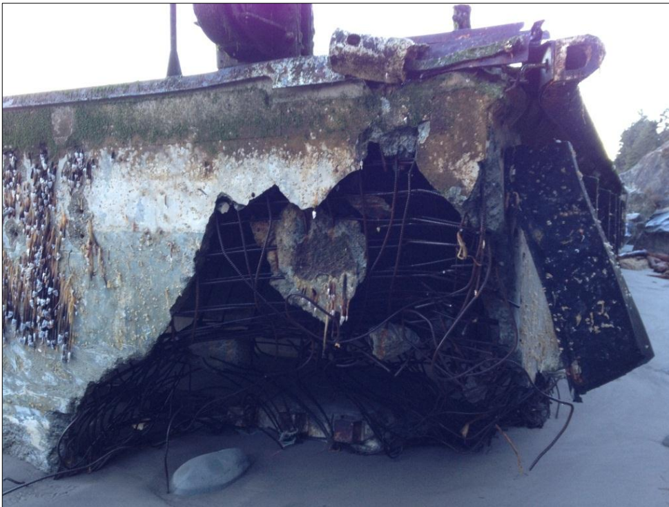
Figure 7: Dock on January 3 rd , 2013, now parallel to the shoreline. Severe damage is visible. (Photo: NPS)
