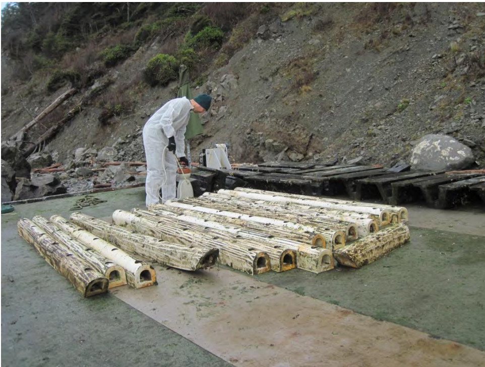
Figure 9: AIS cleanup. Judicious use of bleach on removed fenders and bumpers on Jan 3 (Photo: NPS)
