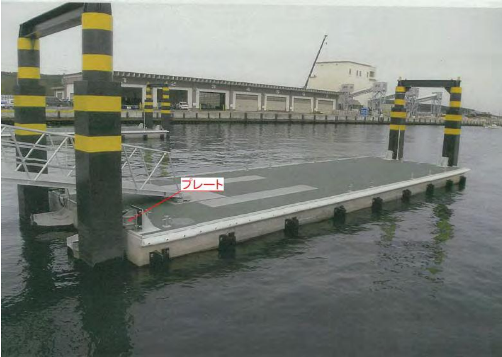
Figure 1: One of floating docks at the port of Misawa (Photo: Port of Misawa)
