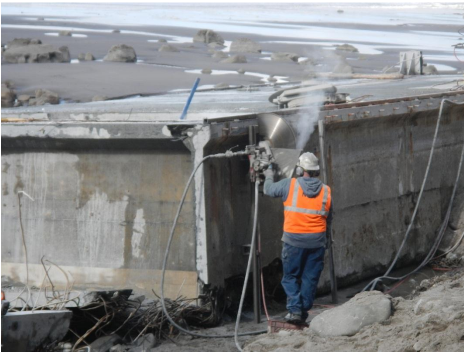
Figure 14: Cutting the dock with a concrete circular saw (Photo: NOAA)
