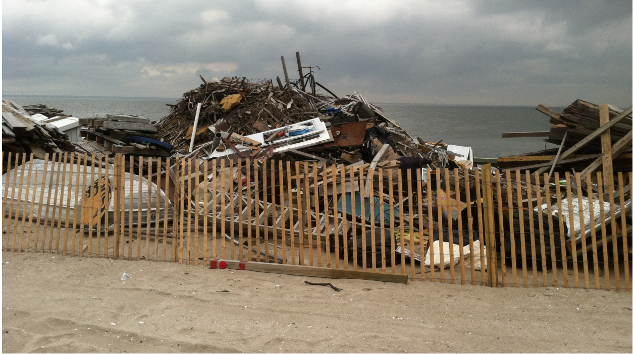
Figure 7: Debris stacked for removal - Fire Island National Seashore.
