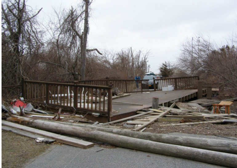
Figure 6: Residential deck and other debris - Gateway National Recreation Area, Jamaica Bay, NY.
