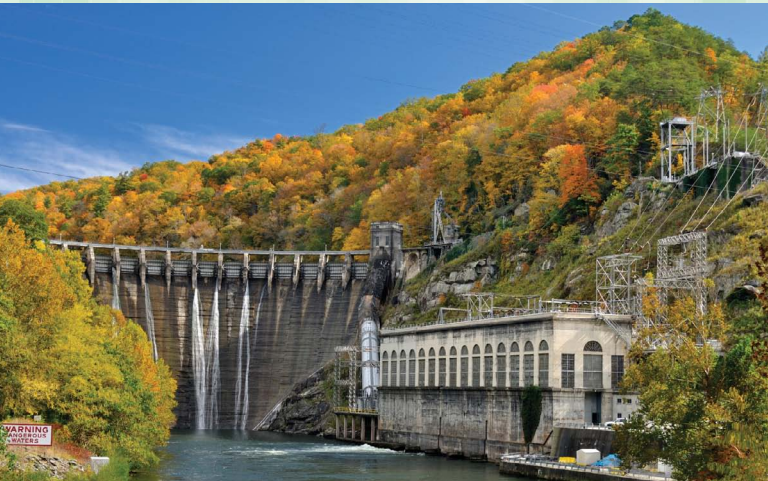
Brookfield Smoky Mountain Project- Cheoah Dam, NC
