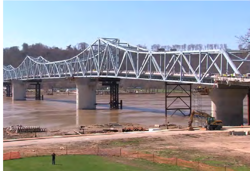
Milton-Madison Bridge slide
