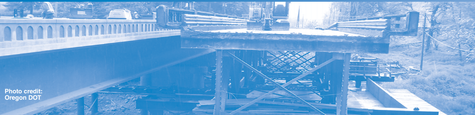
In the Oregon project, the old bridge is the steel truss structure at right, seen after being slid onto temporary piers. The new bridge is at left.
