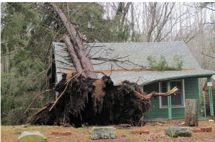
Tree failure resulting in damage to a house in Kennebunkport, ME. (Photo courtesy of USDA Forest Service)
