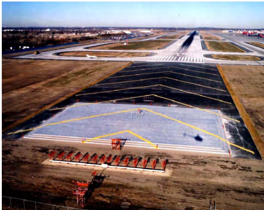
FIG AD 1.1-56 Engineered Materials Arresting System (EMAS)
