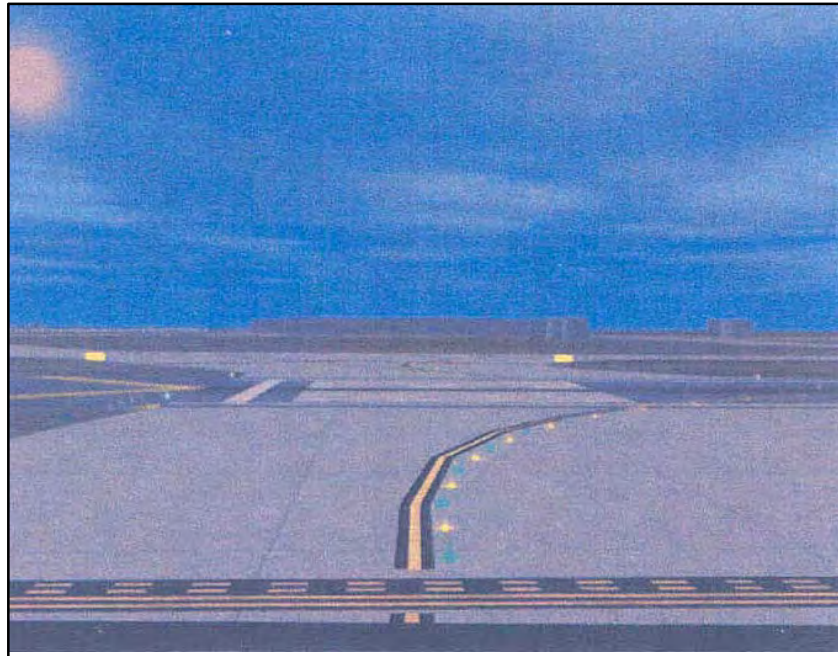
FIG AD 1.1-14 Taxiway Lead-On Light Configuration
