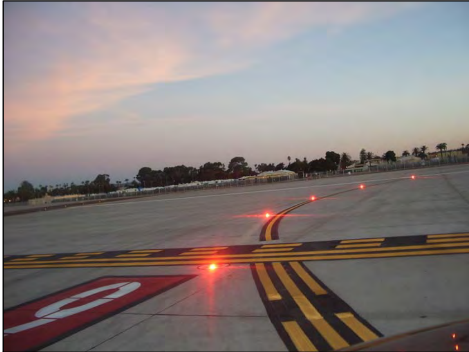
FIGAD 1.1-12 Runway Entrance Lights
