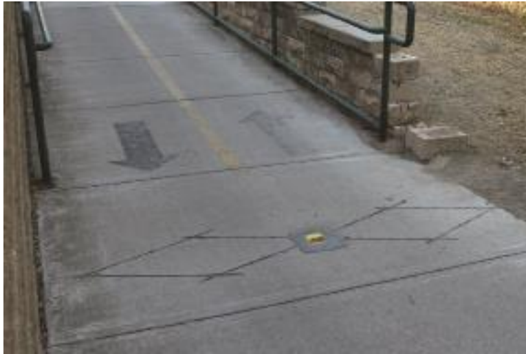
FIGURE 4-3H EXAMPLES OF INDUCTANCE LOOP DETECTOR SHAPES FOR BICYCLIST COUNTING ELONGATED DIAMOND SHAPE: PHOTO
