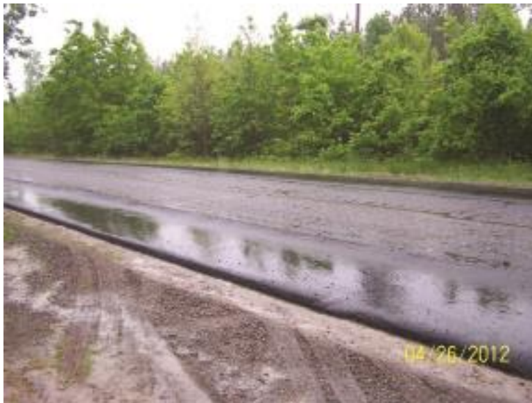
FIGURE E-11 OVERALL SENSORS FACING EAST
