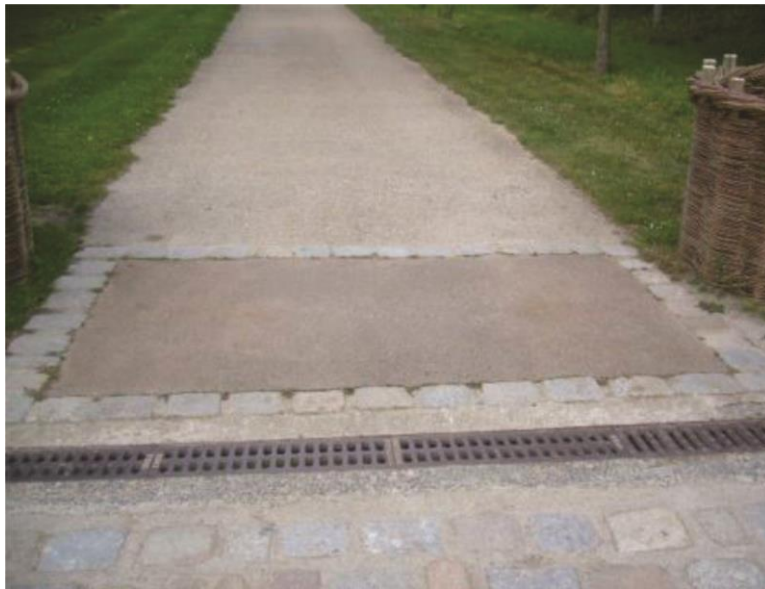
(b) Pressure sensor on paved surface
