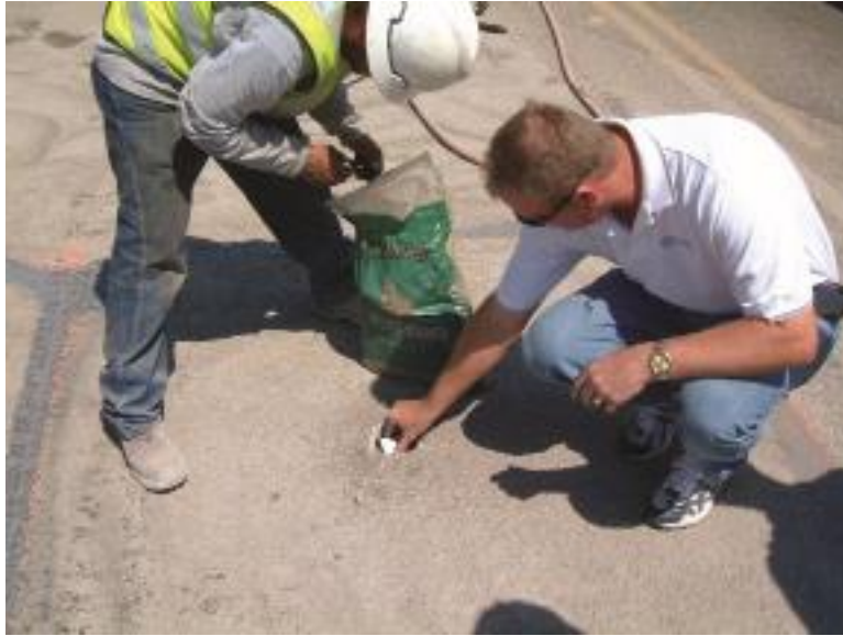
FIGURE 4-7 WIRELESS MAGNETOMETER BEING INSTALLED FOR MOTORIZED TRAFFIC
