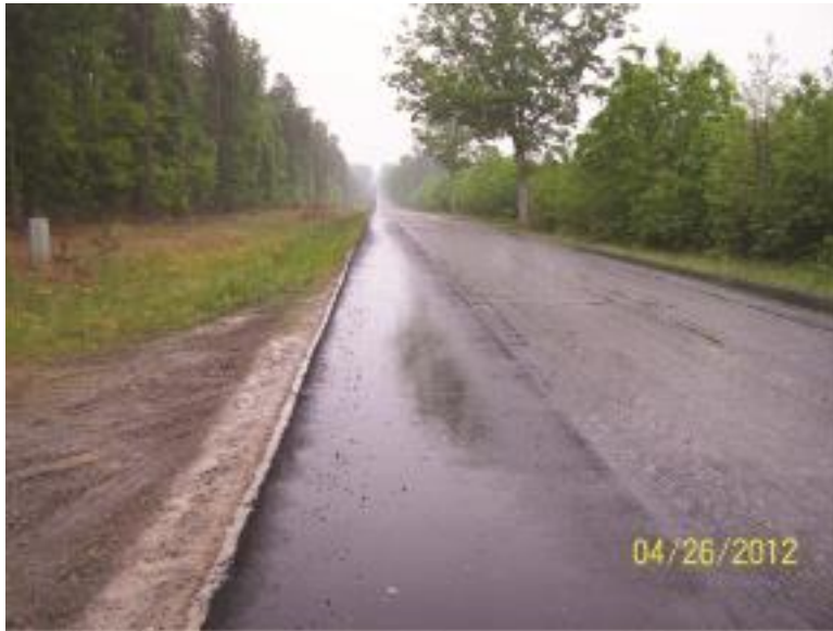
FIGURE E-10 OVERALL VIEW OF ROADWAY FACING EAST
