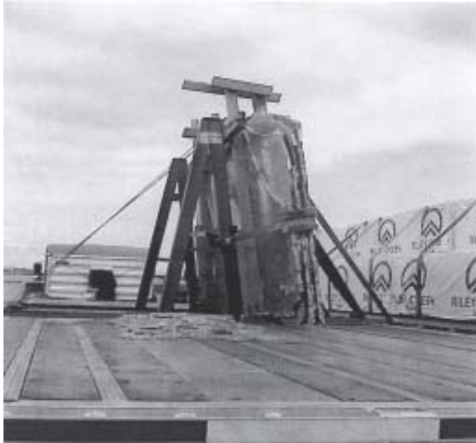
A-frame rack used to transport rock slabs
