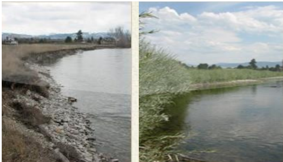
An example of river restoration using conservation practices such as fabric and willow planting. Photo Source: Jeff Tiberi
