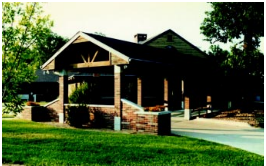
The Butterfield Residential Care Facility has had no recordable injuries or illnesses within the last 3 years. Photo courtesy of Citizens Memorial Healthcare Foundation
