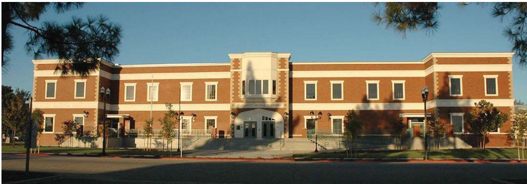
Figure 2: New Flamson Middle School Building (October 2010) Source: Dave Skinner Photography
