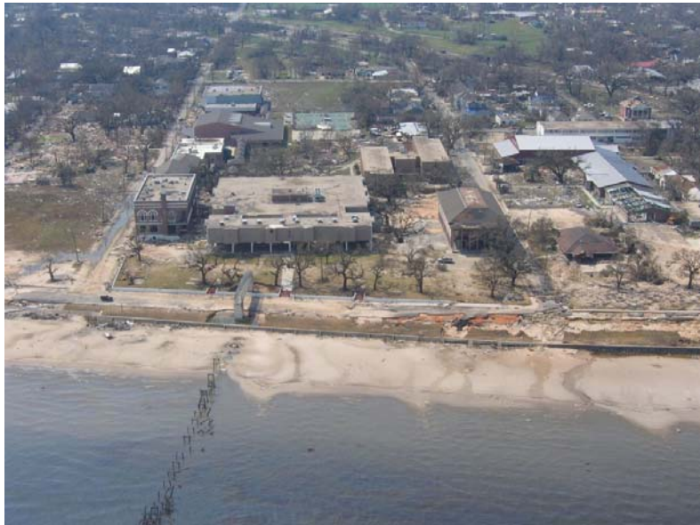
Figure 1: St. Stanislaus College Preparatory – Katrina Damage
