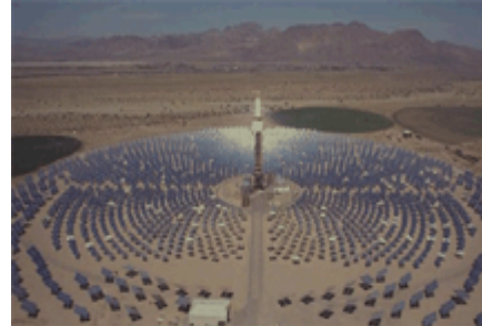
Figure 5.1.2. Power tower solar system (Solar Two).
