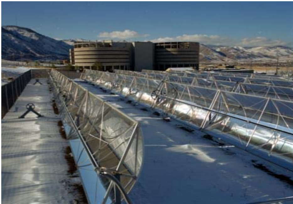
Figure F-4. This 4000 sf solar thermal system is similar to the size and type considered here.
