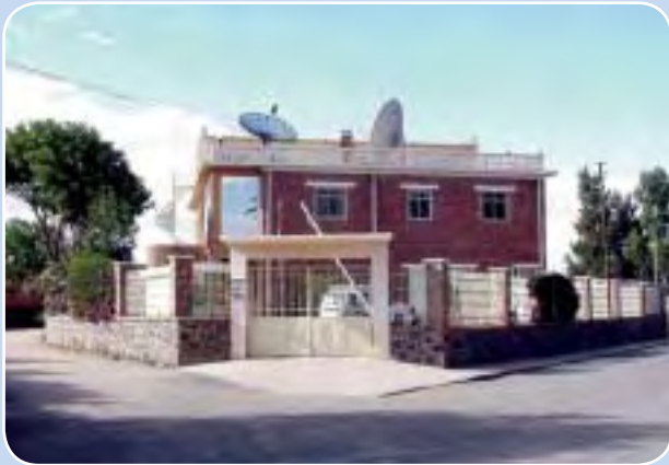
USAID's former office building in Asmara, Eritrea with inadequate setback from street. PHOTO: USAID/OFFICE OF SECURITY (SEC)
