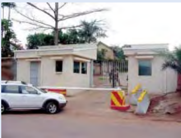
New guard booth with enhanced vehicle screening area.
