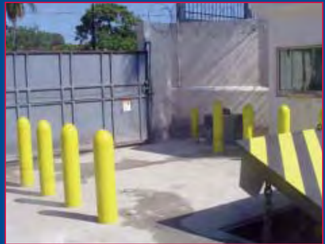
Perimeter gate with anti-ram bollards and vehicle barrier. PHOTO: USAID OFFICE OF SECURITY (SEC)
