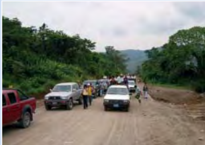
The FBT road rehabilitated with an investment of $25 million, the biggest USAID/Peru grant for one single piece of infrastructure. The “road for development” will facilitate access to markets, new means of passenger transportation, and the integration of this Amazon region with the rest of the country. The immediate impact in people’s life is the reduction in travel time on the Tocache – Juanjui stretch from 16 to four hours. The rehabilitation work emphasized the central stretch of around 90 kms. PHOTO: MABE ARCE, USAID/PERU
