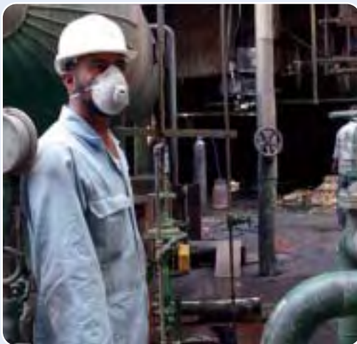
Iraqi workers carry out renovation of the Al-Doura power plant in Baghdad, Iraq. USAID is funding the repair of Iraq's nationwide electrical system.
