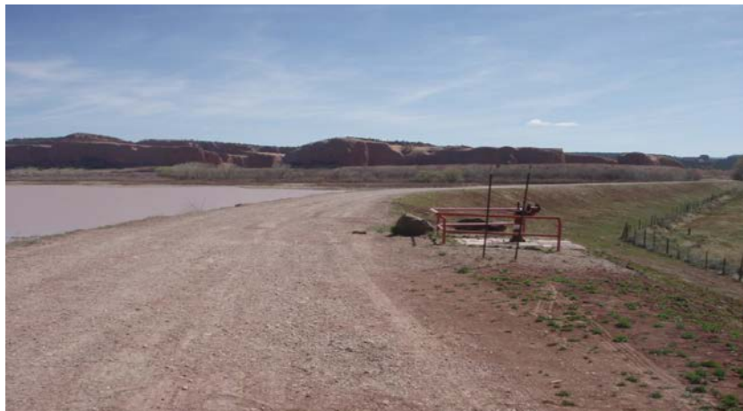
Red Lake Dam, NM
