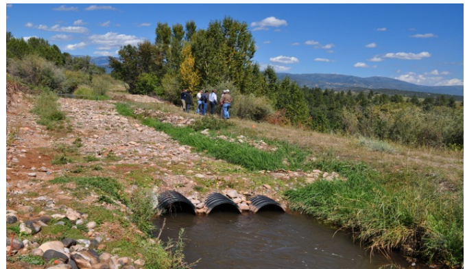
Dr. Morrison Canal, Pine River Irrigation Project, CO
