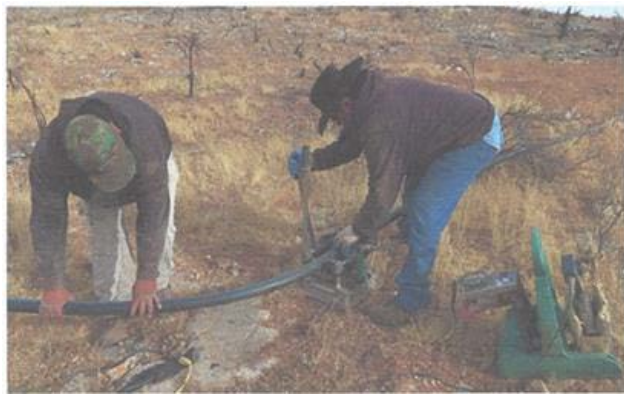
Repairing Hualapai water lines
