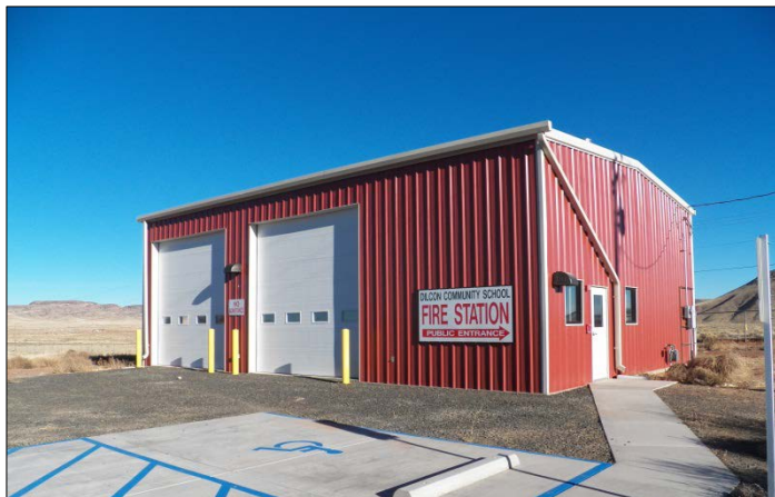
Fire Station at Dilcon Community School in Arizona
