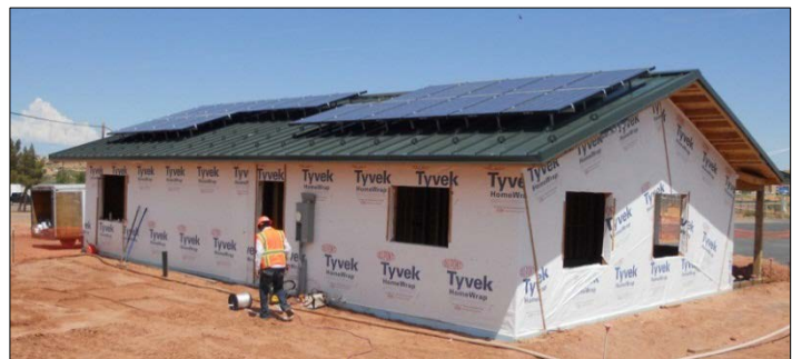
PS&J Quarters under construction in Moencopi, Arizona
