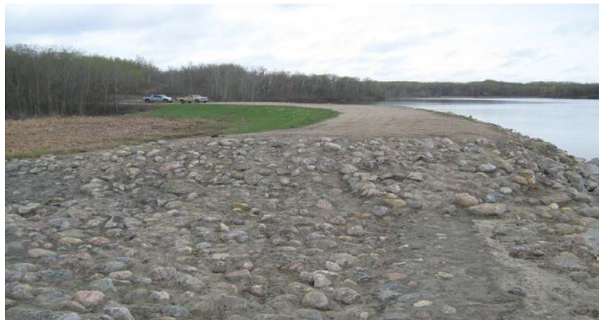
Gordon Dam, ND
