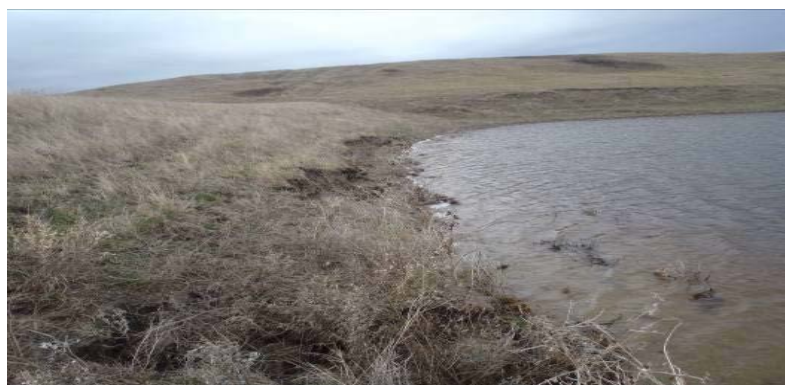
Sully 2 Dam, SD
