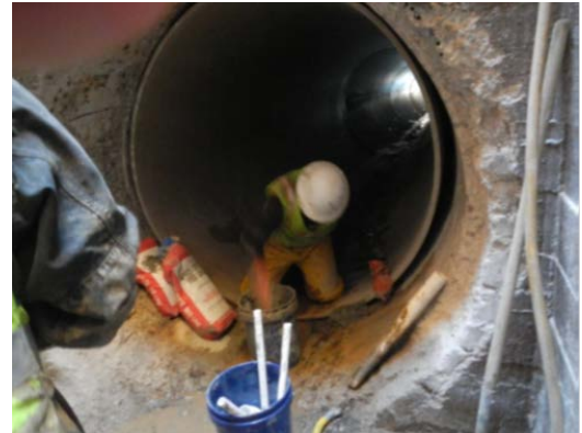
Tyhee Siphon, Ft. Hall Irrigation Project, ID
