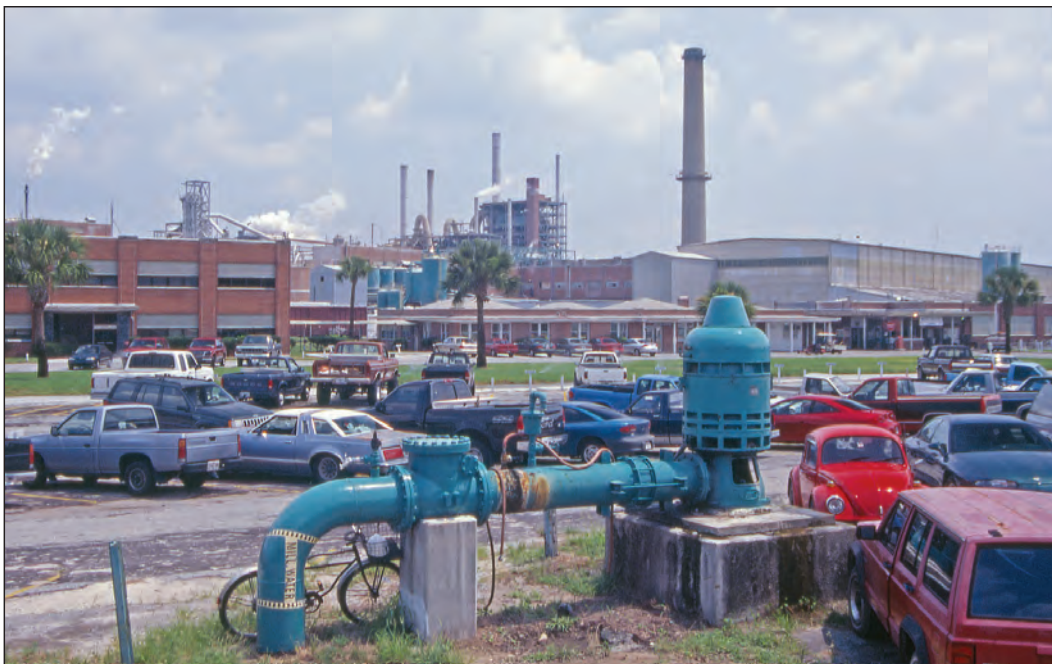
Large capacity well at a paper mill, St. Marys, Georgia. Photo by Alan M. Cressler, USGS.
