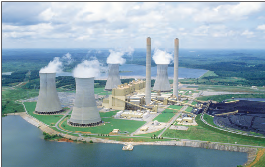
Plant Scherer in Georgia is one of the largest coal-fired thermoelectric power plants in the United States. Photo courtesy of Georgia Power, a Southern Company.
