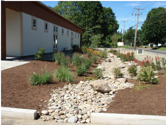
Figure 2-7 Bioretention cell at a commercial site Photo courtesy Berkshire Design Group
