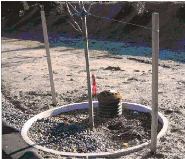
Figure 2-12 Tree box filter
