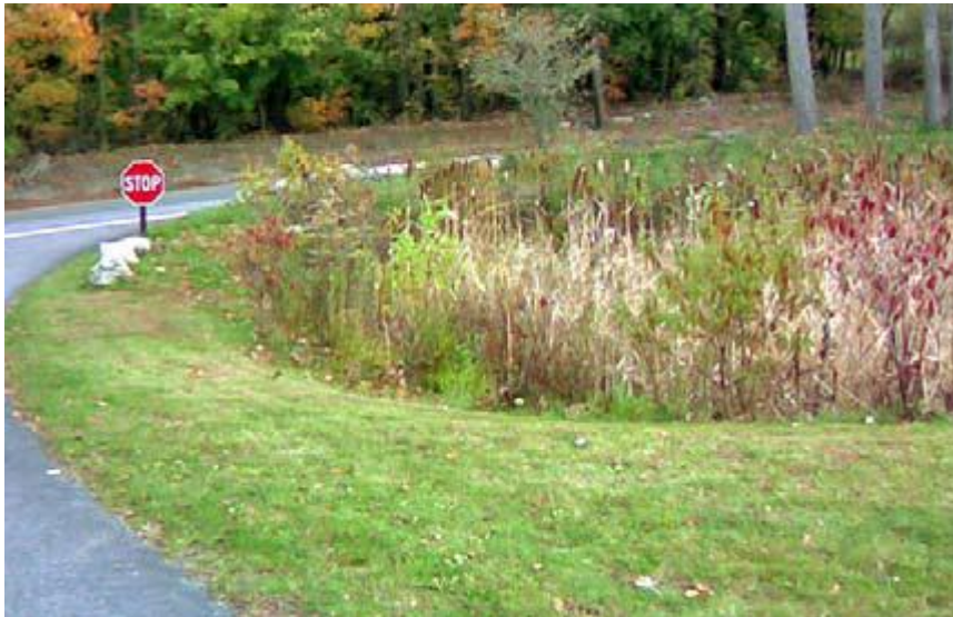
Figure 2-4 Constructed stormwater wetland
