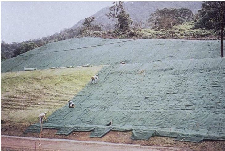
Figure 3-1 Geotextiles used for stabilizing a hill
