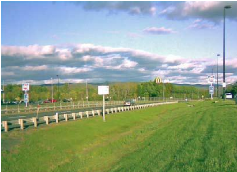
Figure 2-1 Dry water quality swale
