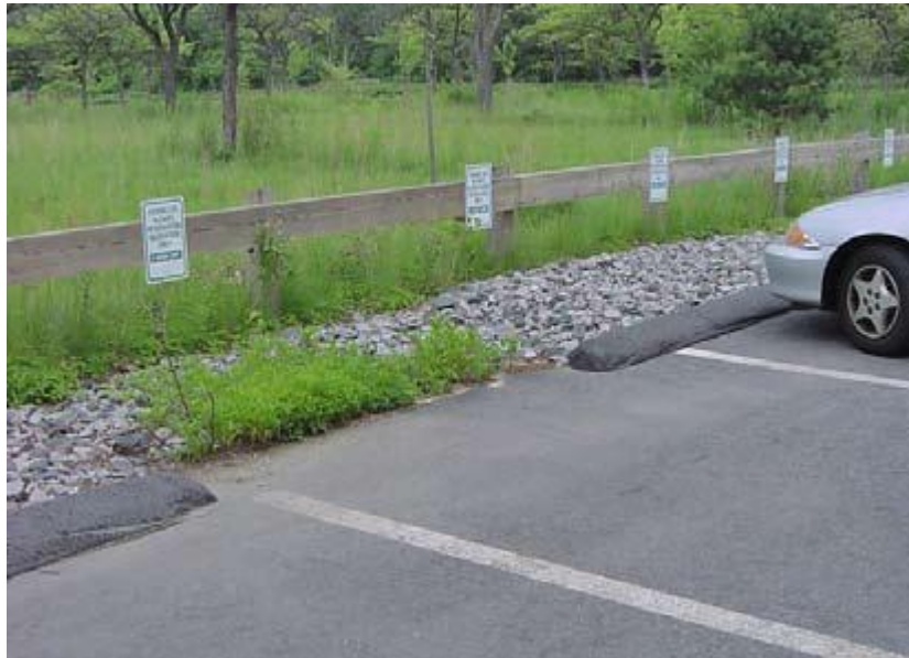
Figure 2-2 Vegetated filter strip
