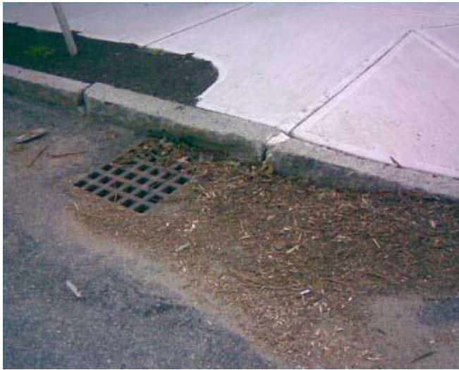
Figure 2-17 Deep sump catch basin inlet
