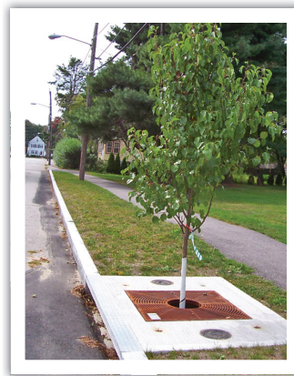
Tree filter box in Milton, MA. Neponset River Watershed Association
