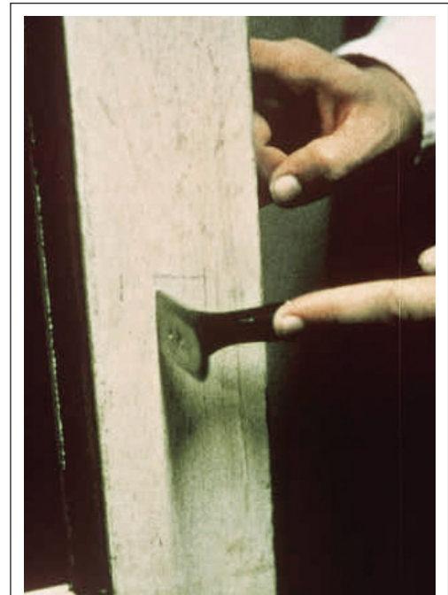
FIGURE 7.4 Preparing to take a paint-chip sample for laboratory analysis.
