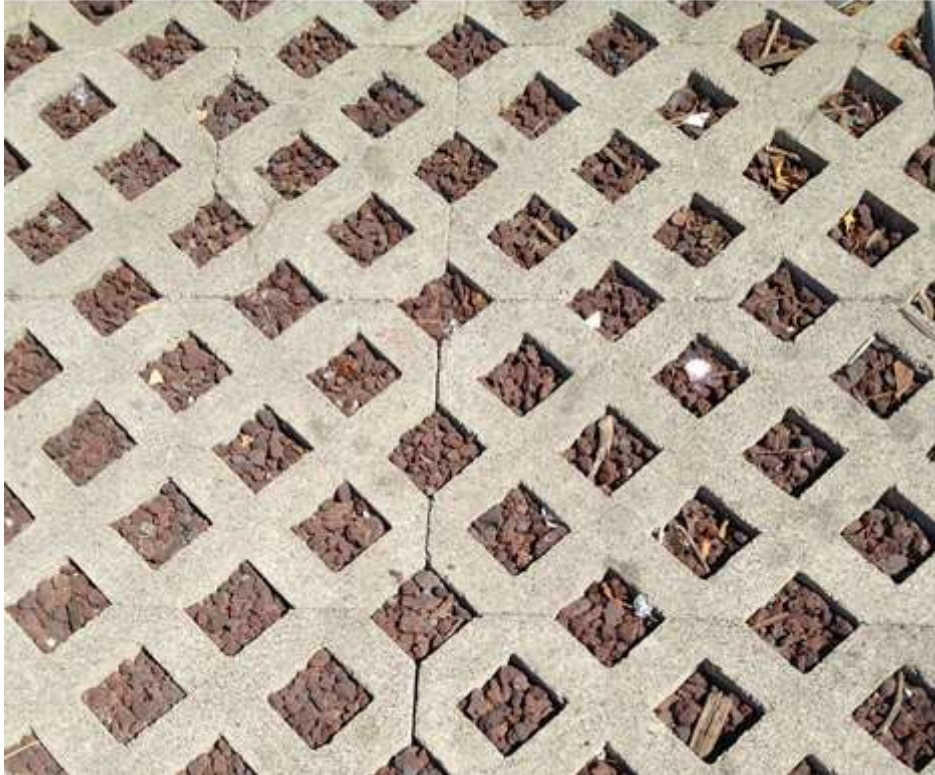
Figure B-3-8. Example of CGPs with volcanic rock bedding course.
