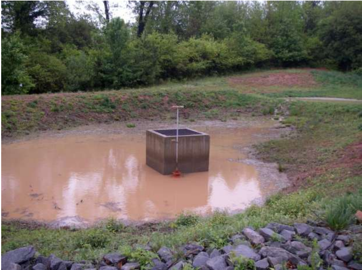
Figure B-7-10. Dewatering intake in a detention facility (similar design applies to stormwater wetlands).
