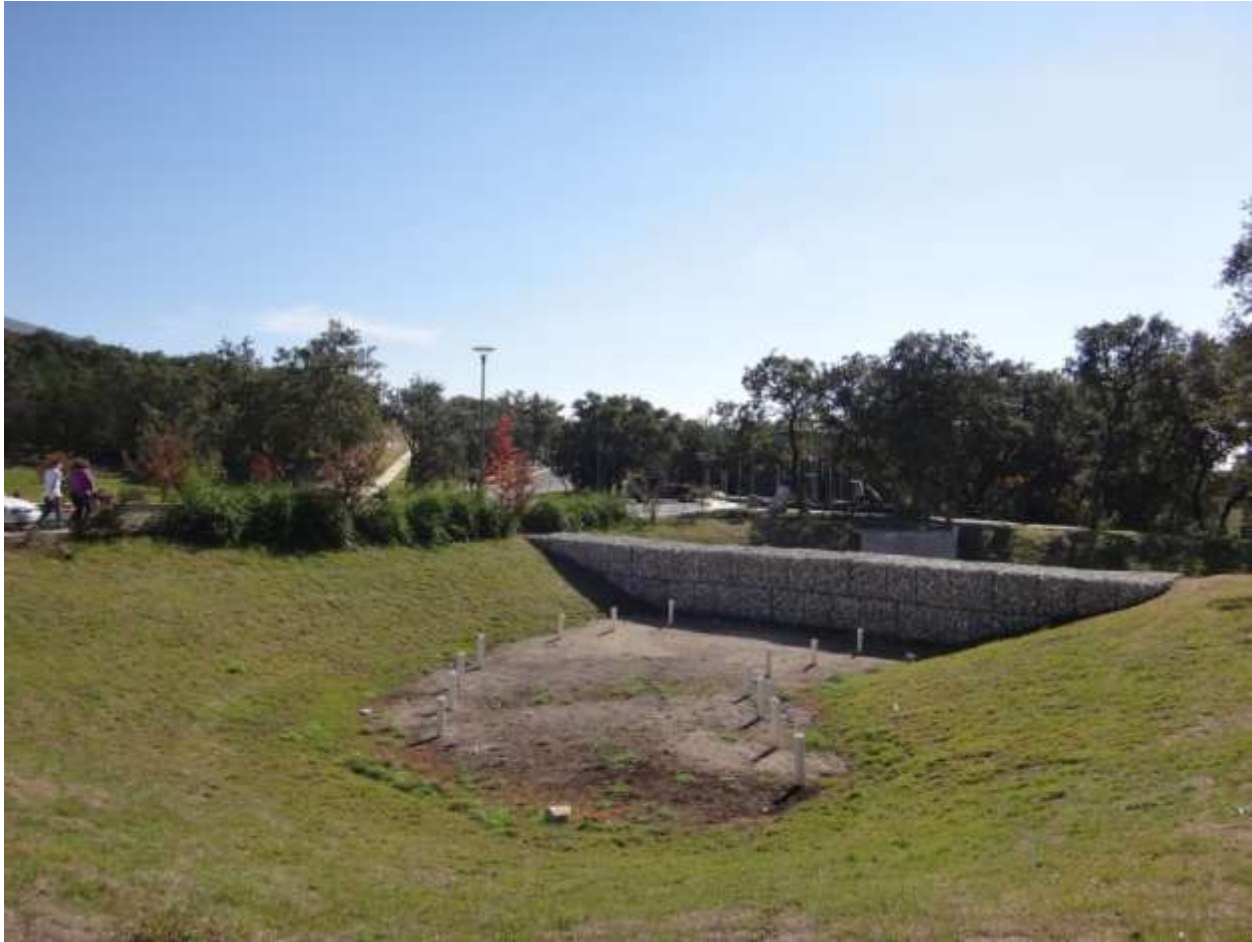
Figure B-6-1. Surface sand filter.
