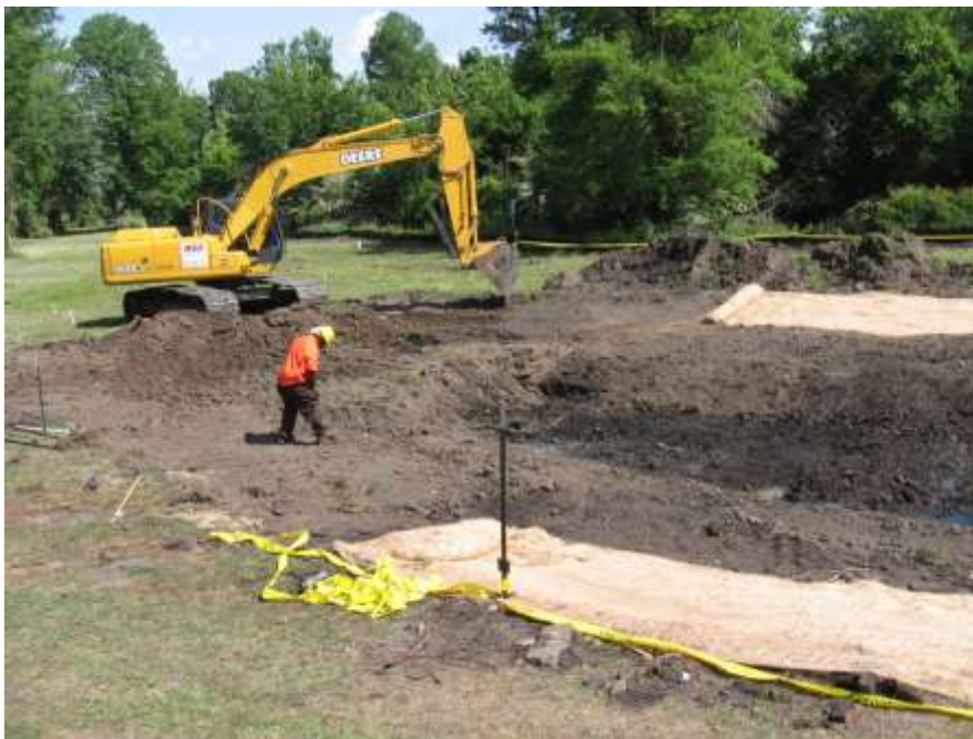
Figure 4-4. Heavy equipment (especially wheeled equipment) should be operated outside the excavated area to prevent compaction.
