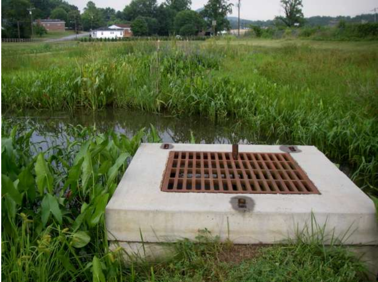
Stormwater wetland in Lenoir, North Carolina. Source: Tetra Tech, Inc.
