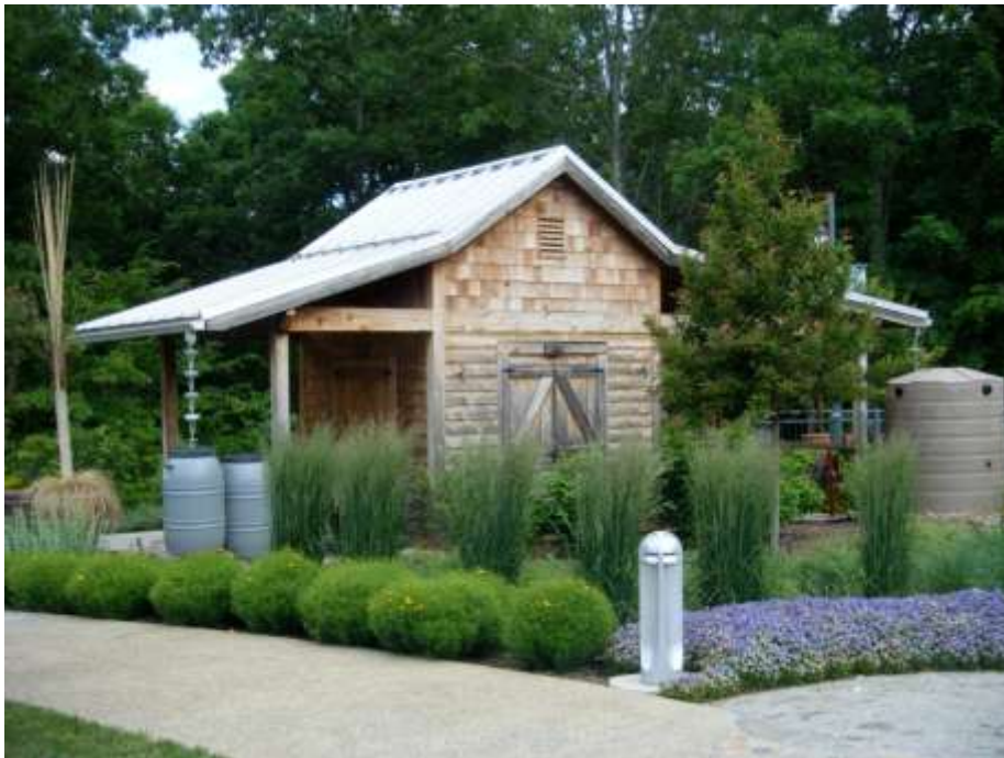
Asheville, North Carolina Source: Tetra Tech Figure 3-26. Rain barrels adequately sized for contributing roof area.
