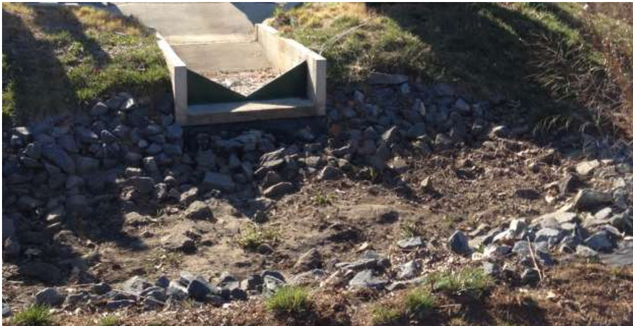
Figure 4-15. Inlet curb cut with a v-notch weir.
