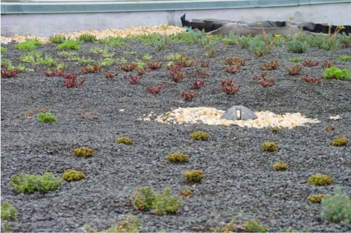
Figure 4-13. White gravel indicates a no plant zone for a green roof.
