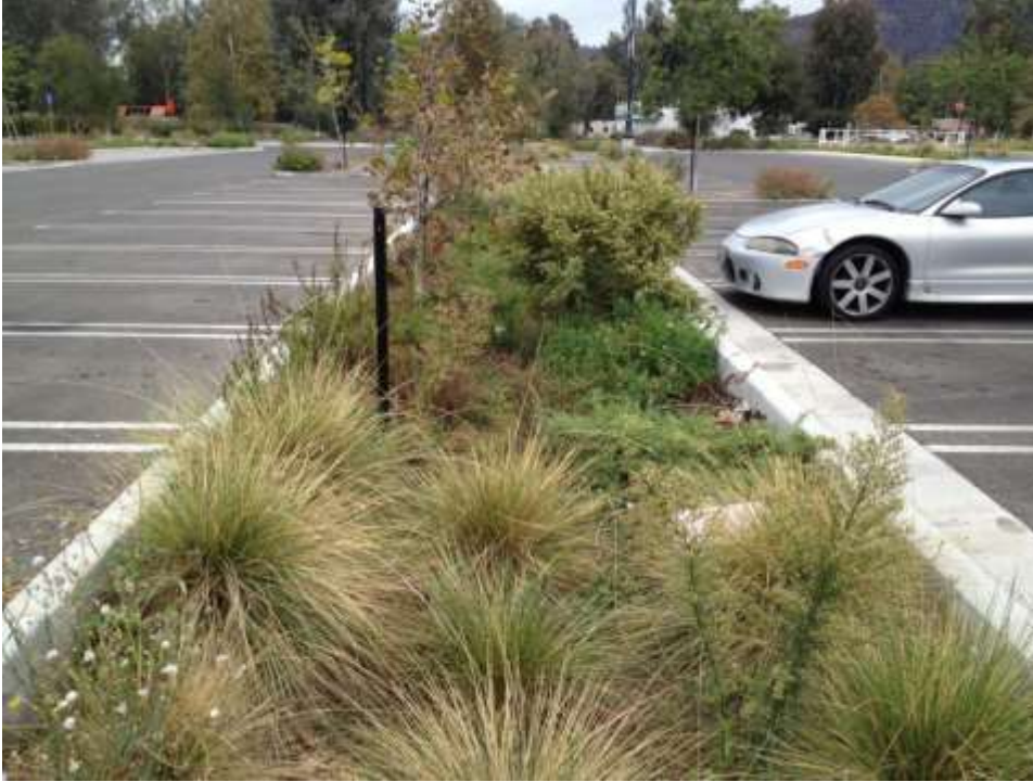
Figure 3-3. Parking lot bioretention area.
