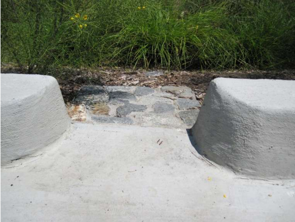
Figure B-11-2. A typical curb cut.
