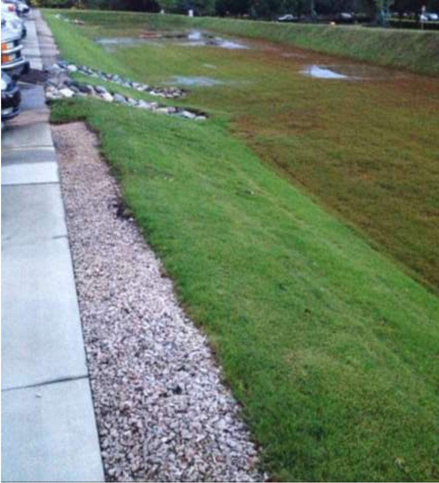
Figure 3-30. Vegetated filter strip surrounding a bioretention area in a parking lot.
