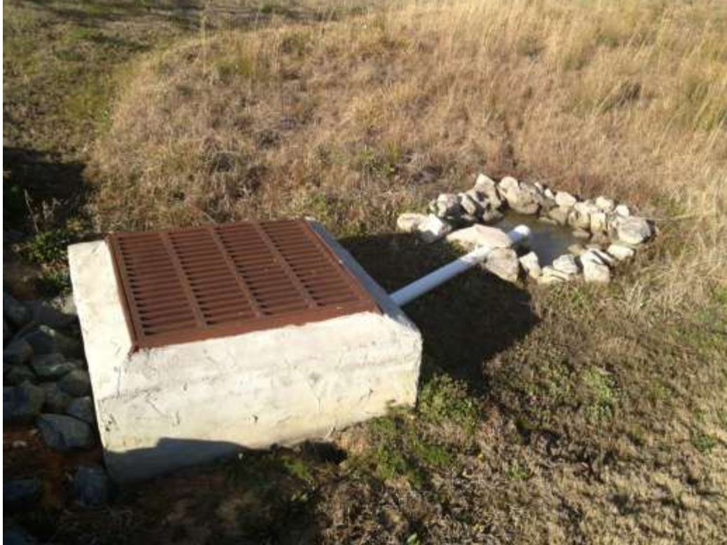
Figure B-7-7. A downturned inlet pipe with an orifice extends into a deep pool in a small stormwater wetland.
