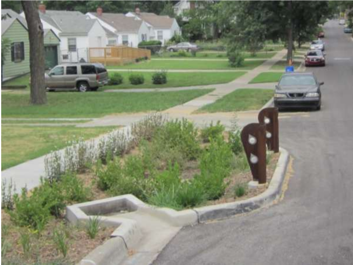
Figure 3-6. Bioretention in a pop-out. A curb cut is provided at the upslope end of the pop-out to accept runoff from the gutter.
