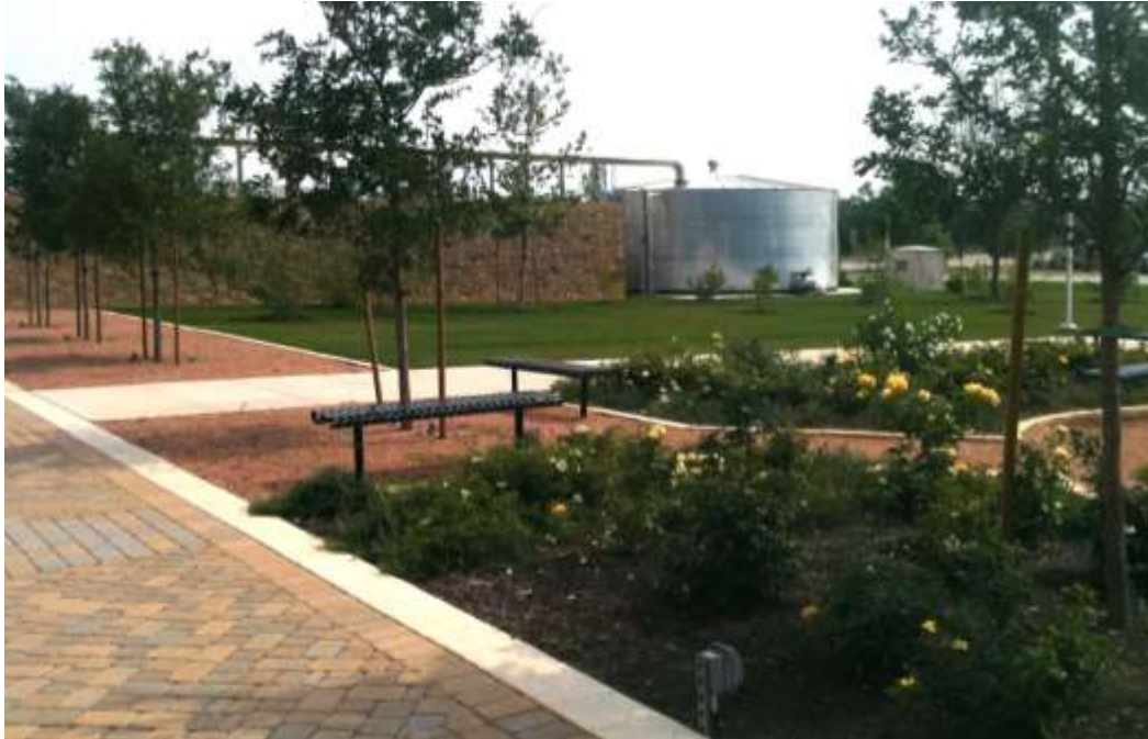
Texas A&M University at San Antonio, San Antonio, Texas. Source: San Antonio River Authority
