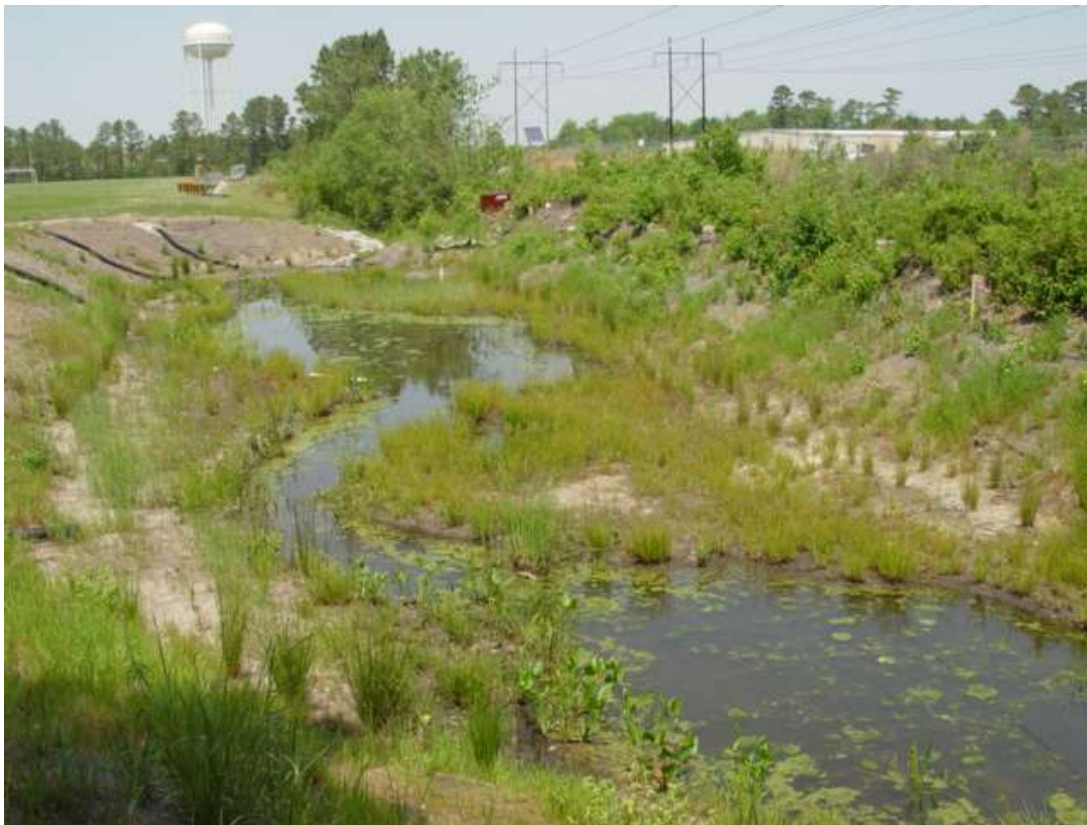
Wilmington, North Carolina. Source: Tetra Tech.
