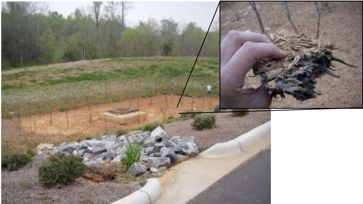
Figure 4-1. Example of a bioretention area installed before permanent site stabilization with the inset photo showing the clay layer clogging the mulch surface.
