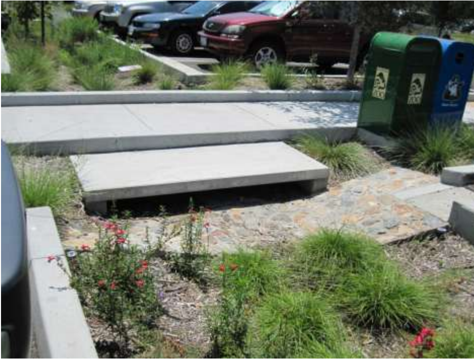
Figure B-1-7. Inlets stabilized with mortared cobble.
