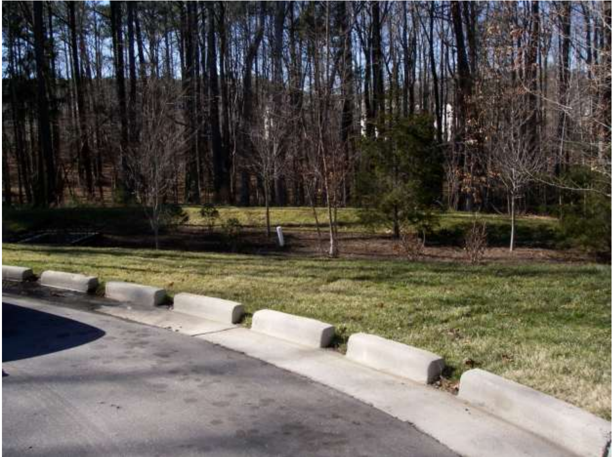
Figure 3-29. Vegetated filter strip that pretreats roadway runoff.
