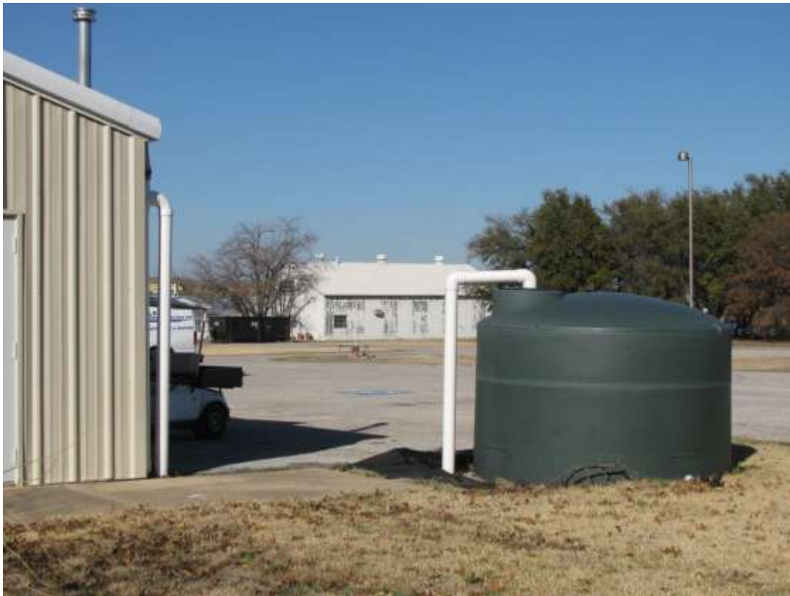
Figure B-8-9. Cistern with a wet conveyance inlet configuration.
