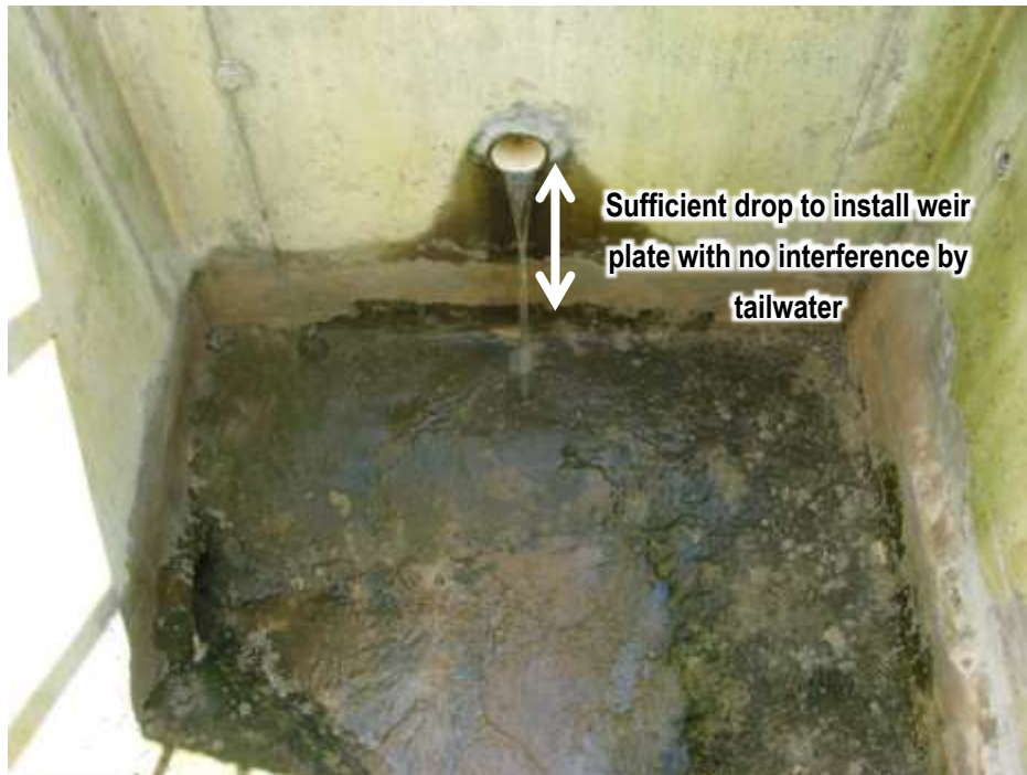
Figure 4-18. Example of a bioretention underdrain outlet with sufficient drop to install a flow monitoring weir without encountering tailwater.
