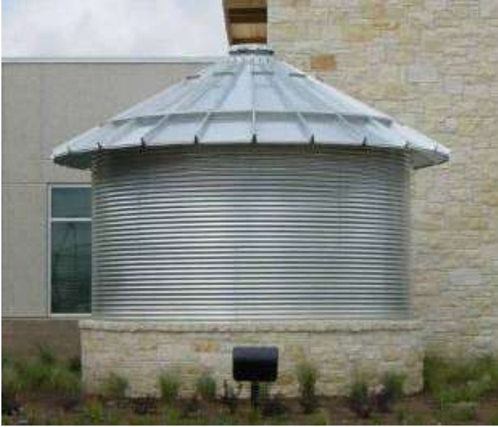
Figure B-8-3. Cistern greater than 2,000 psi on a concrete foundation.
