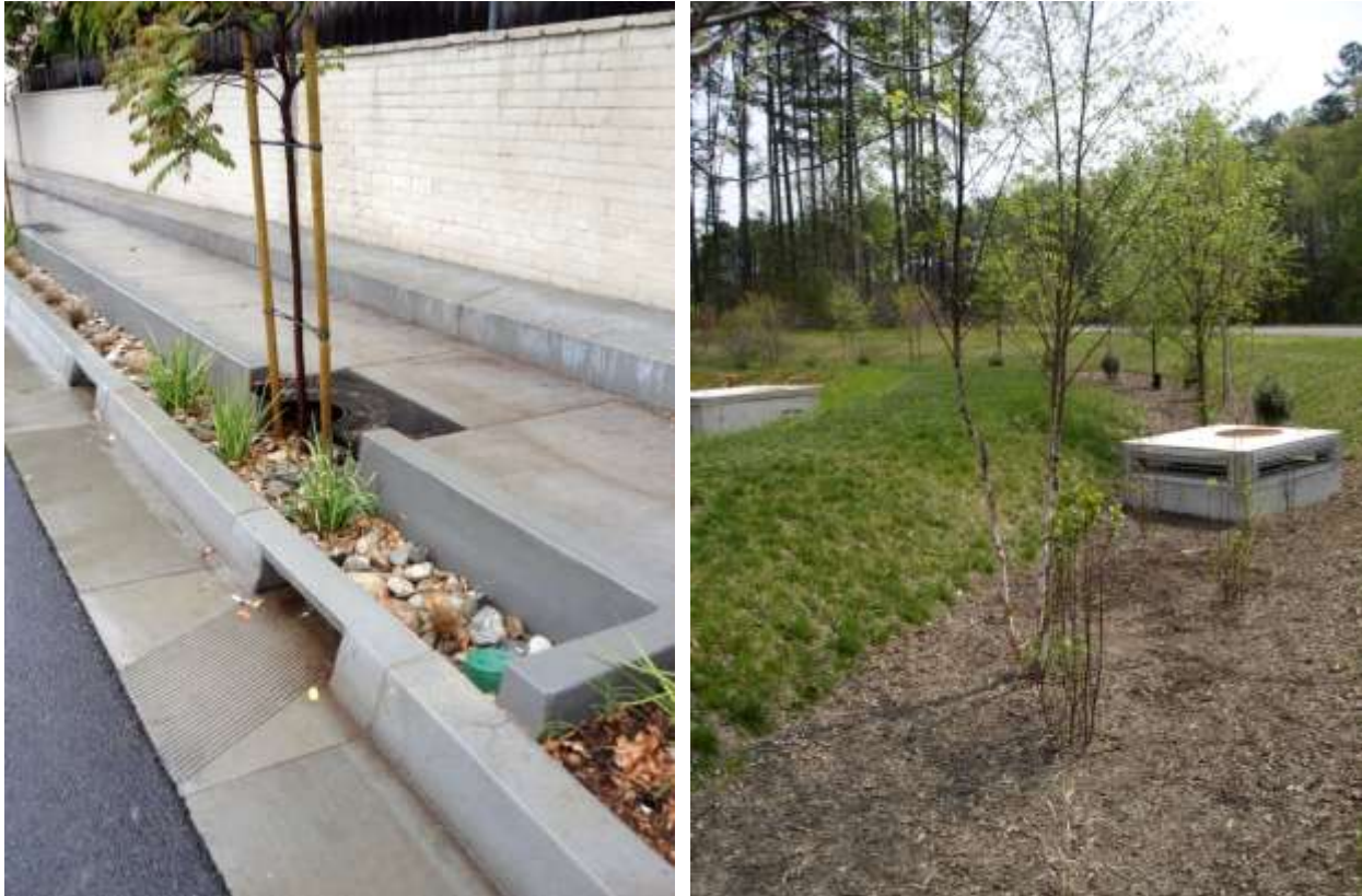
Figure B-2-6. Left: An offline bioswale along the road right of way (excess flow bypass along gutterline). Right: An online bioswale with an overflow outlet structure along a roadway and parking lot (this practice is used in a treatment train with an adjacent detention basin).
