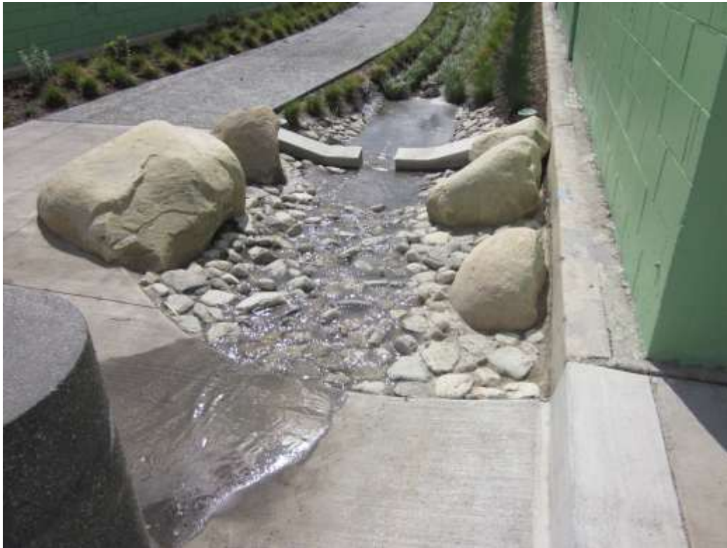
Figure B-1-6. Inlet and pretreatment provided by mortared cobble forebay and energy dissipater.
