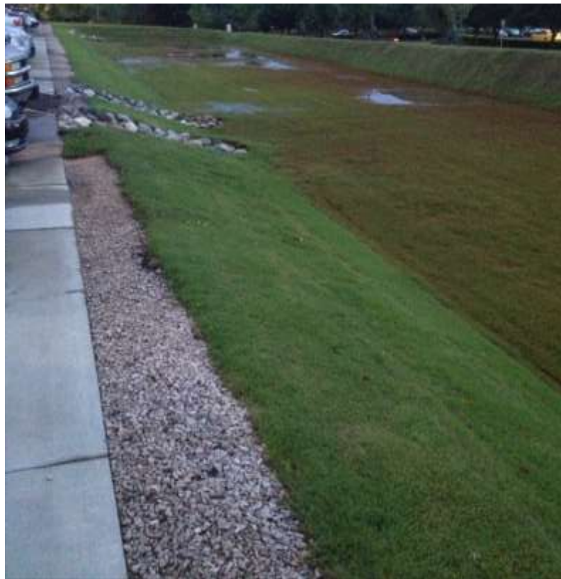
Figure 3-1. Treatment train featuring a vegetated filter strip pretreating runoff before entering a grassed bioretention area.
