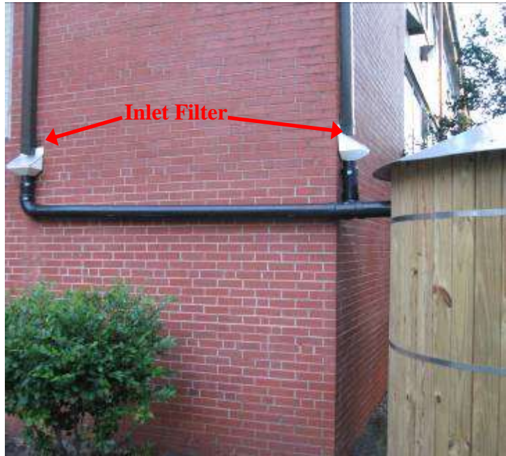
Wilmington, North Carolina. Source: Tetra Tech
