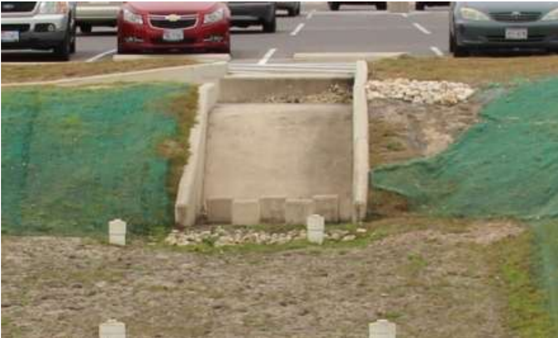
Figure B-11-8. Concrete energy dissipater.
