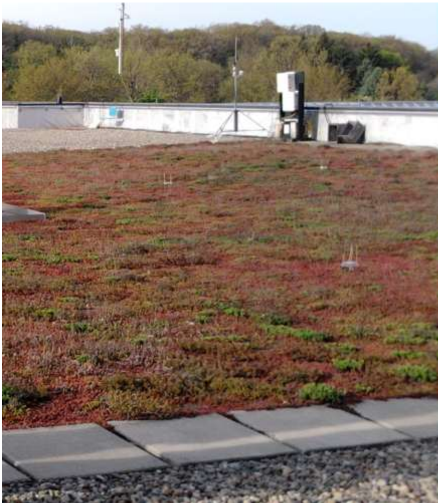
Figure B-5-1. Example of an extensive green roof.
