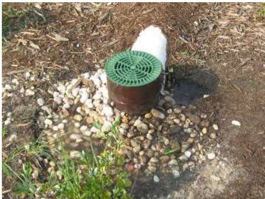
Figure B-11-9. Upturned roof downspout energy dissipater.
