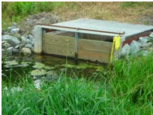
Figure 4-11. Outlet varied with weir boards.
