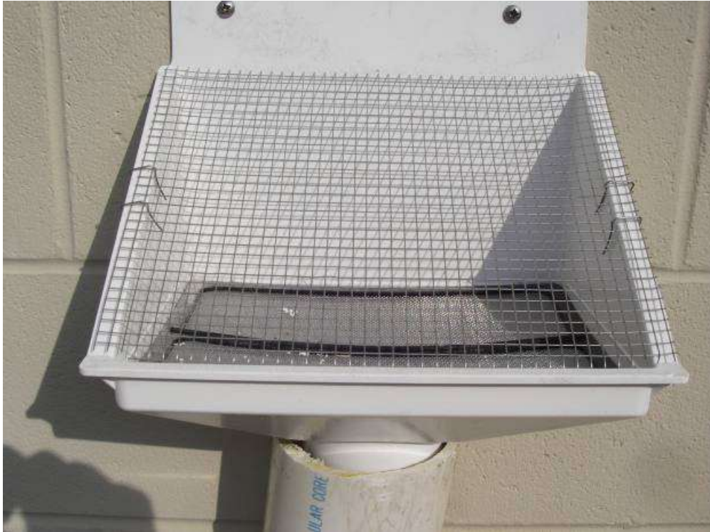
Figure B-8-12. Flow-through inlet filter.
