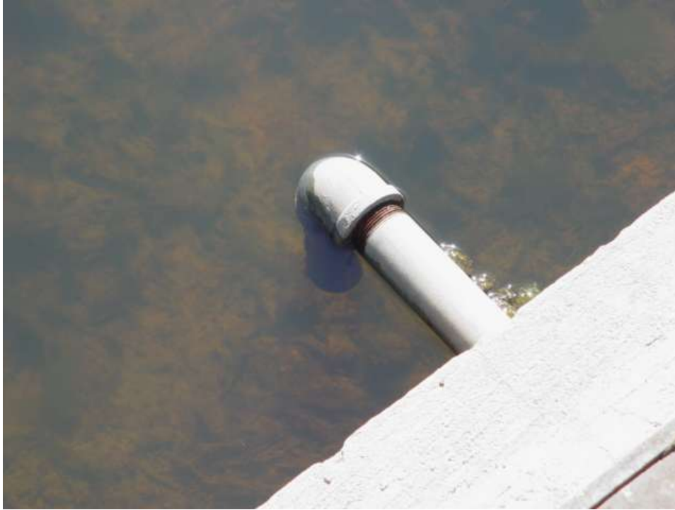
Figure B-11-15. Drawdown pipe with a downturned elbow.
