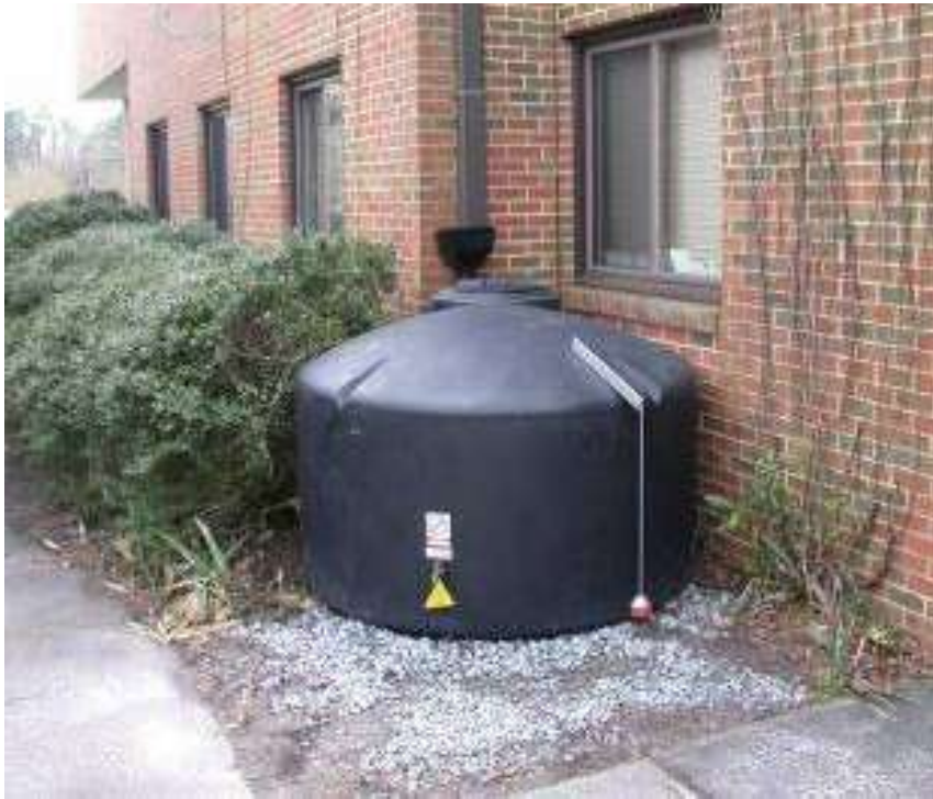
Figure B-8-2. Cistern less than 2,000 psi on a gravel foundation.
