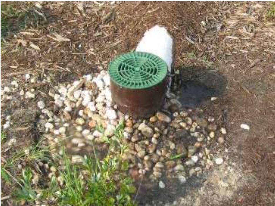
Figure B-1-8. Upturned inlet from rooftop bubbles up diffusely onto gravel pad.
