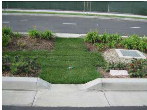
Figure B-11-4. Curb cuts and vegetated filter strip for a roadside bioretention area.
