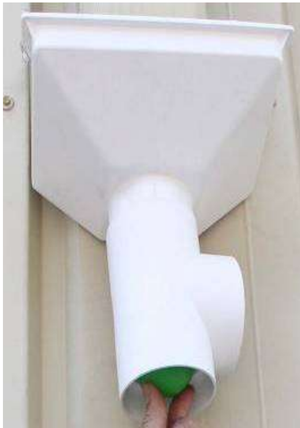
Figure B-8-14. Valve for a first-flush diverter.
