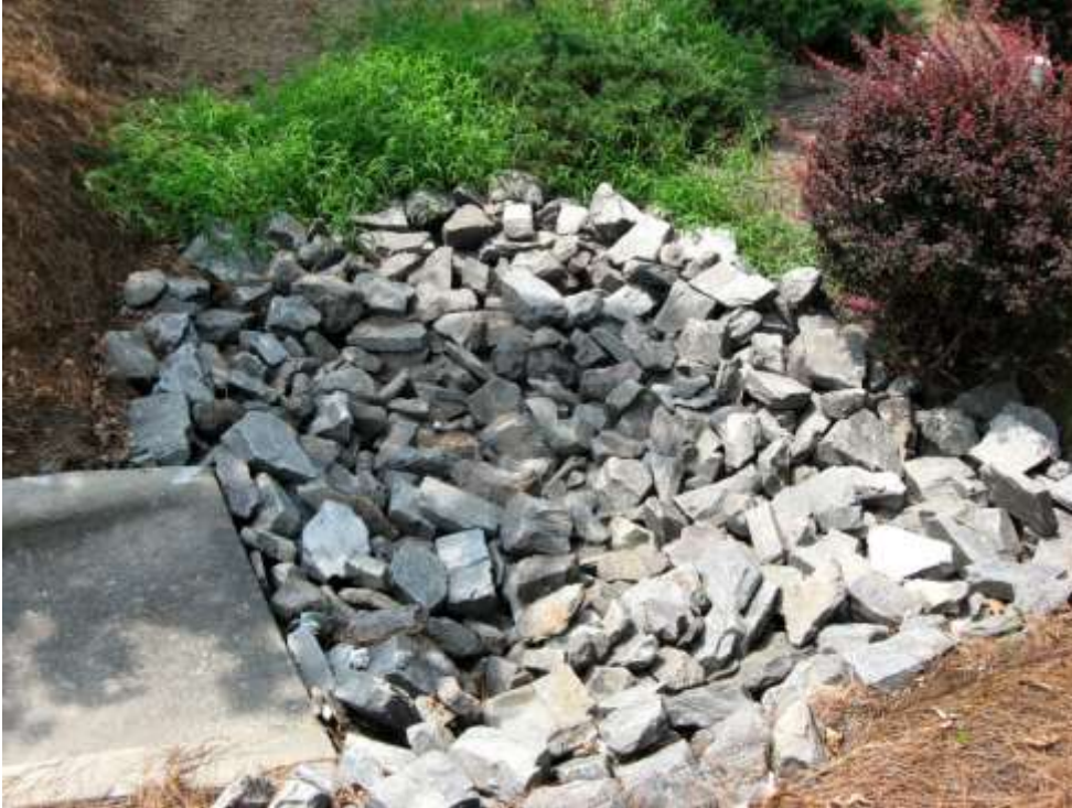
Figure B-11-7. Stone flow dissipater/forebay.
