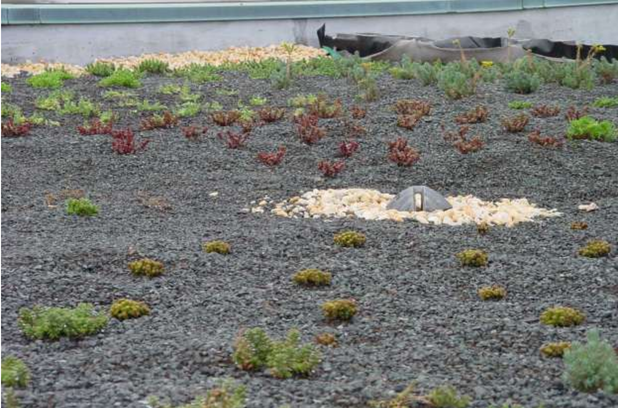
Figure B-5-4. Light-colored gravel delineates the no-planting zone for maintenance personnel.
