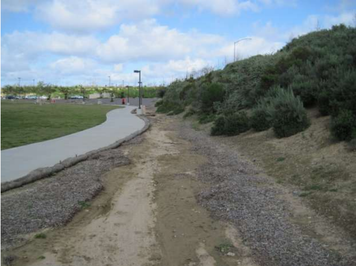
Figure 4-8. Erosion caused by excessive flows in a bioswale.
