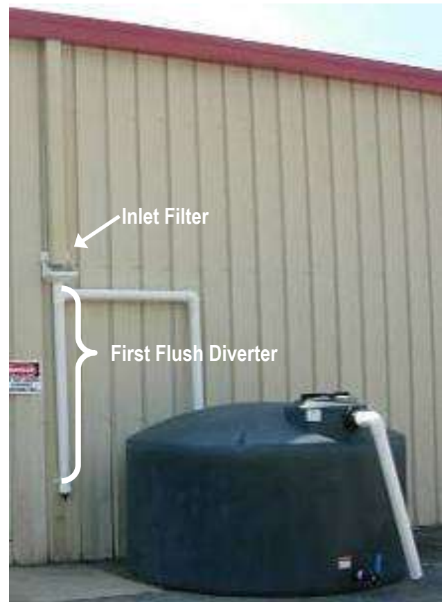
Figure B-8-15. First-flush diverter configuration.
