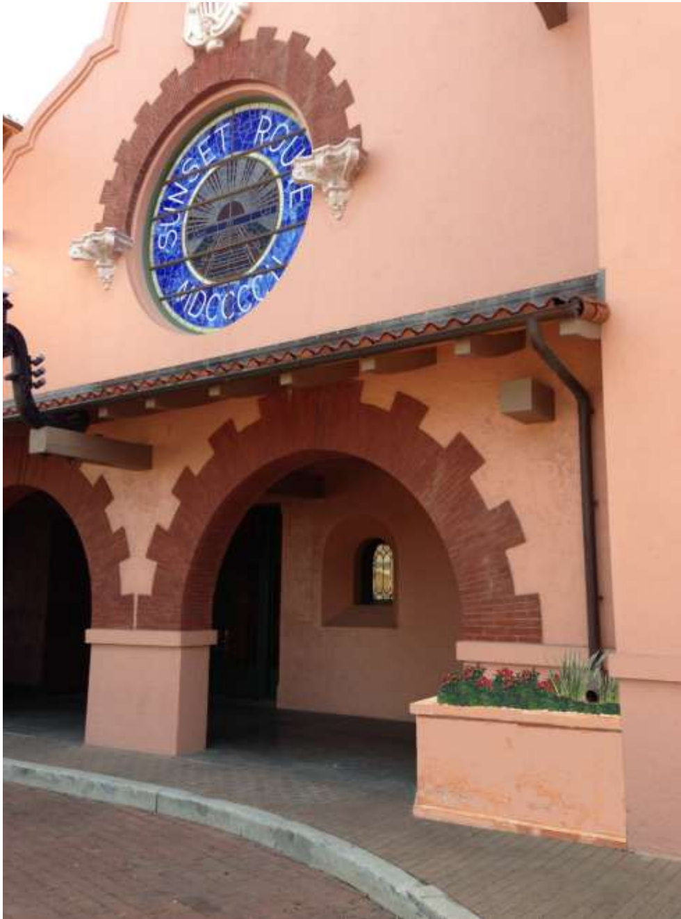
Planter box retrofit to treat rooftop runoff at Sunset Station, San Antonio, Texas (rendering)
