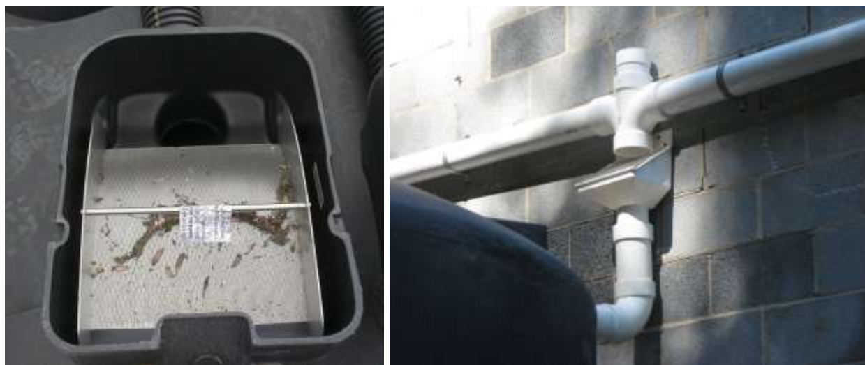
Figure 4-10. Self-cleaning inlet filters.
