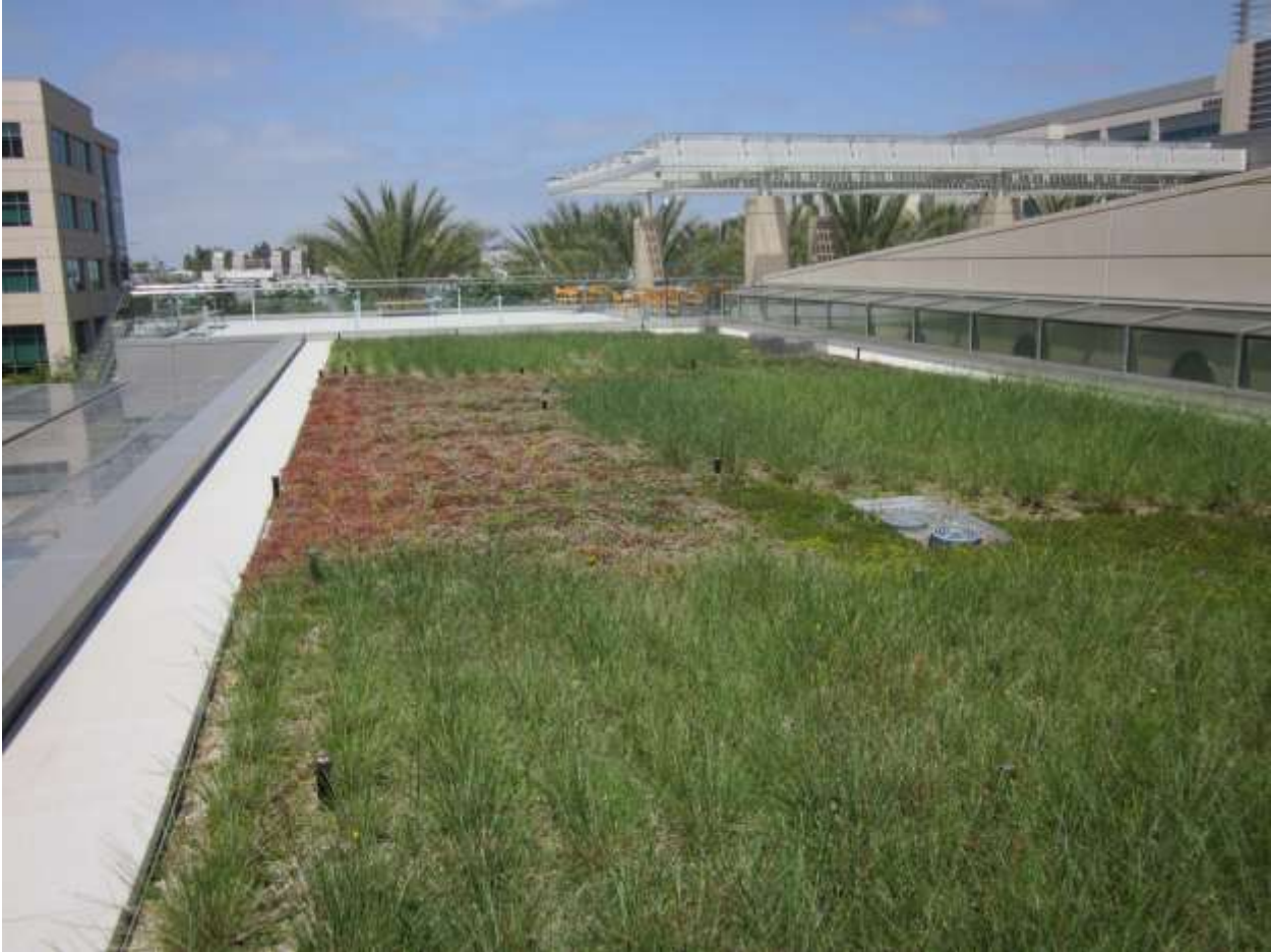
County Offices, San Diego, California. Source: Tetra Tech
