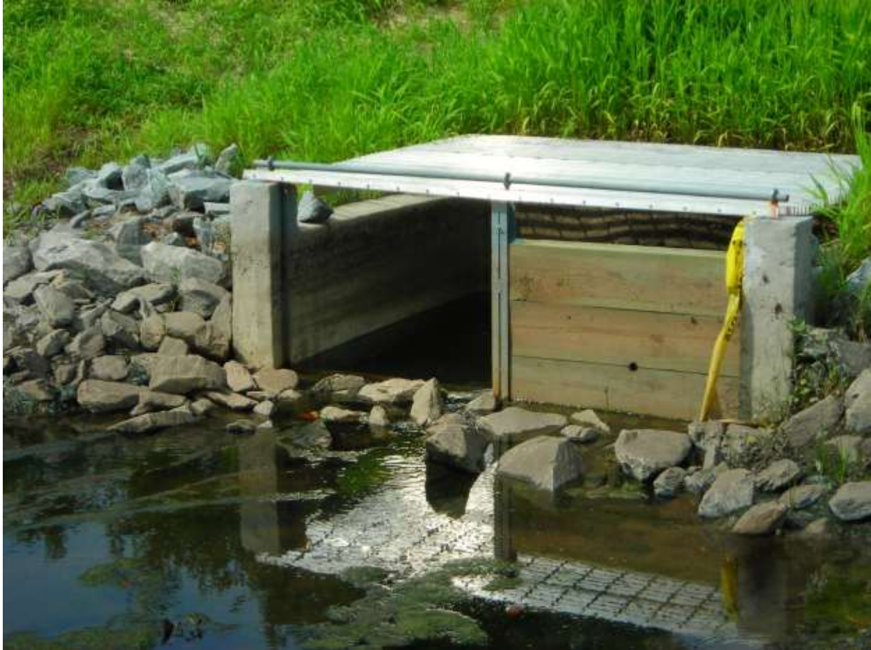
Figure B-7-9. A flashboard riser allows adjustment of water level during plant establishment and for maintenance.
