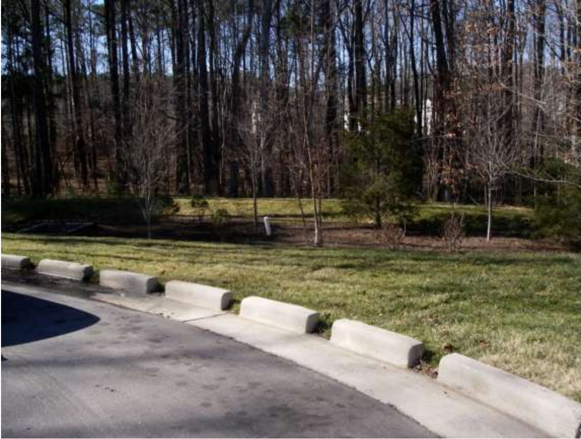
Figure B-11-4. Curb cuts and vegetated filter strip for a roadside bioretention area.
