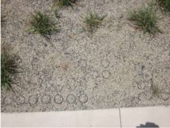
Figure 3-12. Permeable pavement fire access lane.
