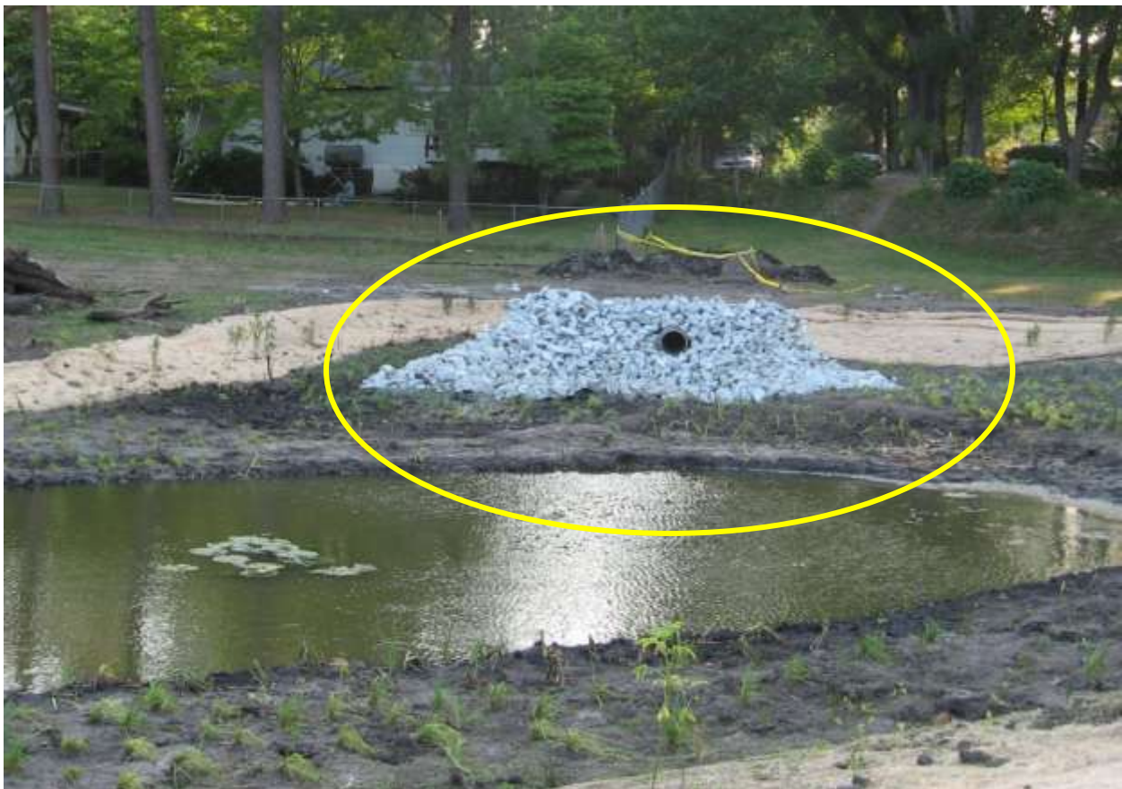
Figure B-7-2. Forebay visible in a newly planted wetland.
