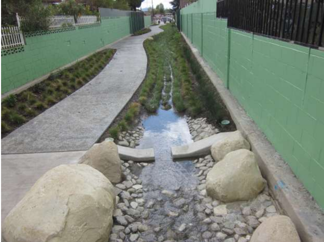
Bioswale at Elmer Avenue, Los Angeles, California. Source: Tetra Tech
