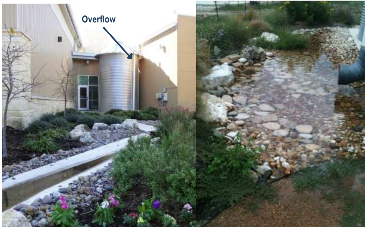
Figure B-8-18. Left: A channel directs overflow away from building. Right: A cistern overflows to an adjacent bioretention area.
