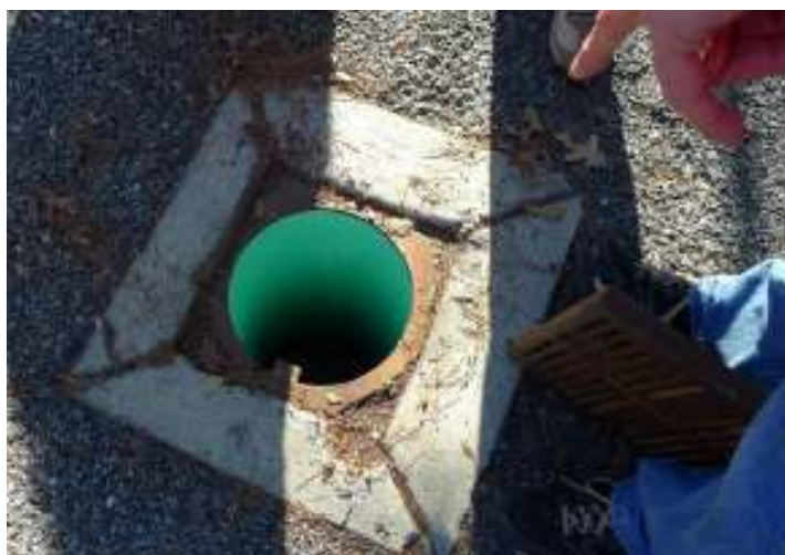
Figure B-3-13. Observation well installed in permeable pavement.
