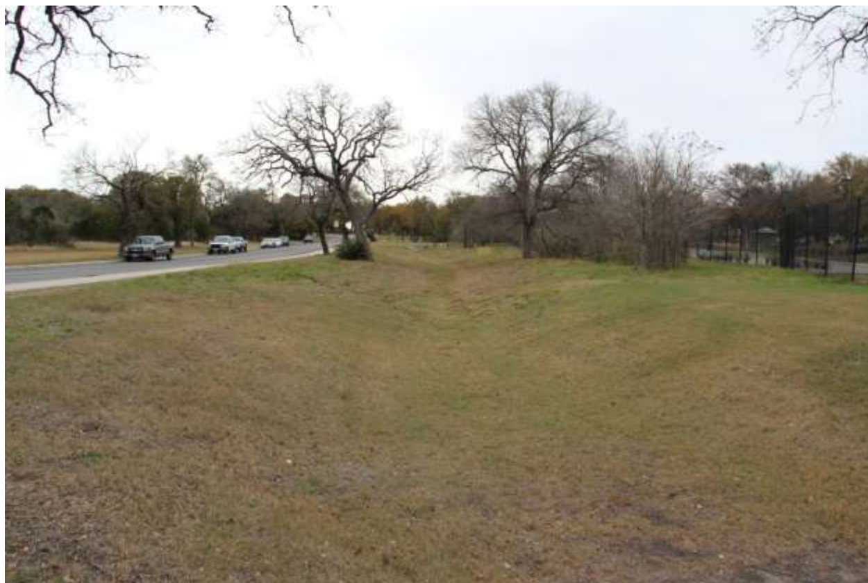
Figure 3-28. Roadside vegetated swale.
