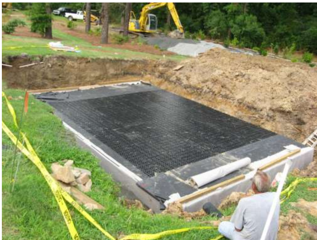
Figure 3-24. Below ground cistern.
