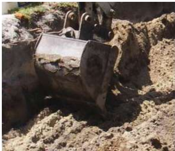
Figure 4-5. For infiltrating practices, mitigate subsoil compaction by ripping grade to a depth of 12 inches.
