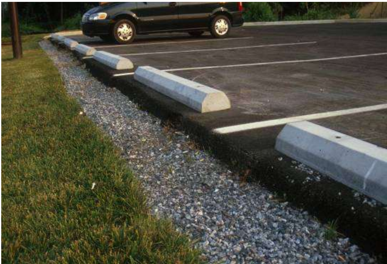
Louisburg, North Carolina. Source: NCSU B AE
