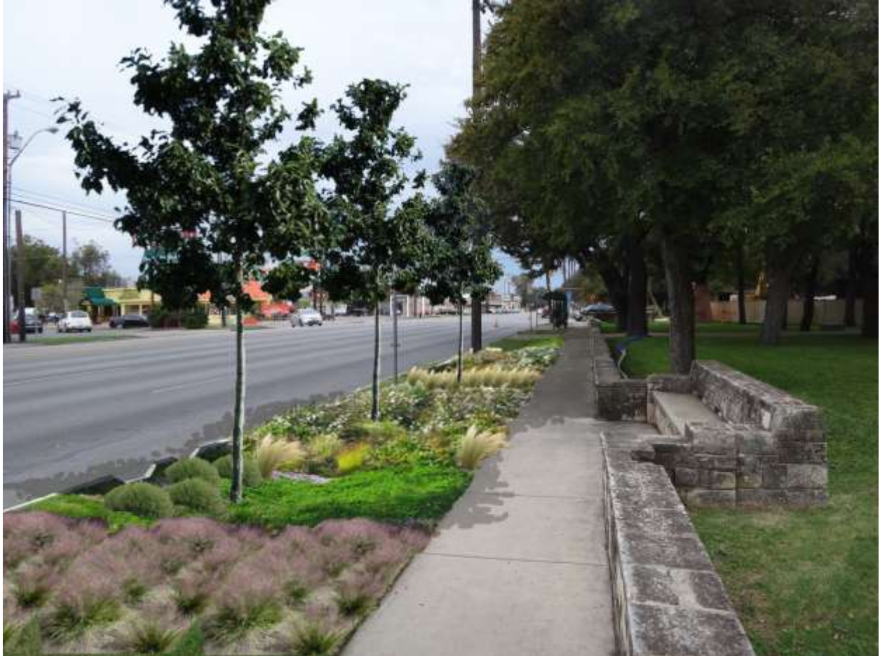
Bioretention in the right-of-way on Broadway Street, Witte Museum, San Antonio (rendering). Runoff is intercepted from the street through curb cuts and from the sidewalk by sheet flow.
