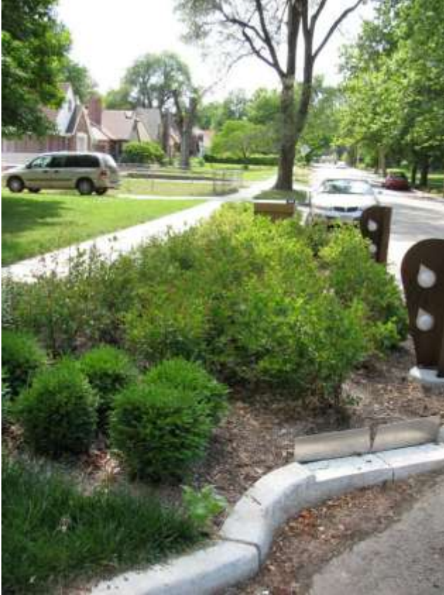
Figure 4-16. Outlet of a roadside bioretention pop-out equipped with a V-notch weir for flow monitoring.
