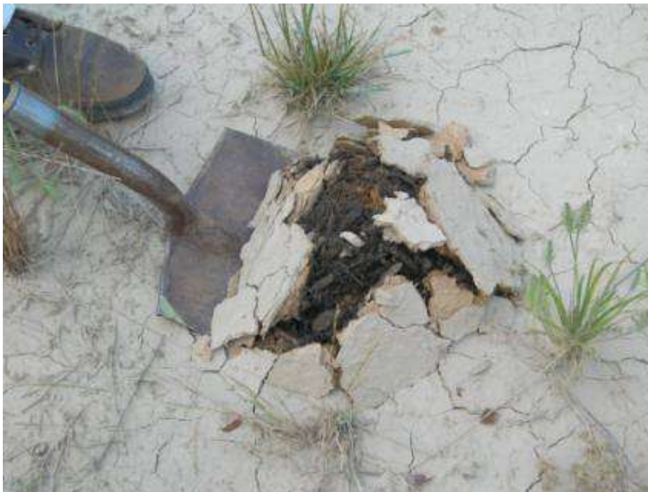
Figure 4-6. Bioretention area clogged with sediment.
