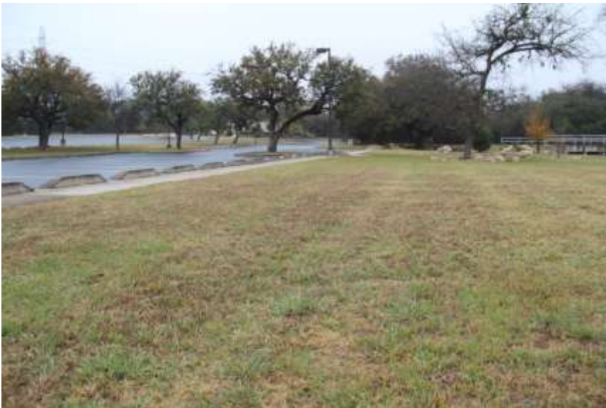
Figure 3-31. Vegetated filter strip next to a parking lot.
