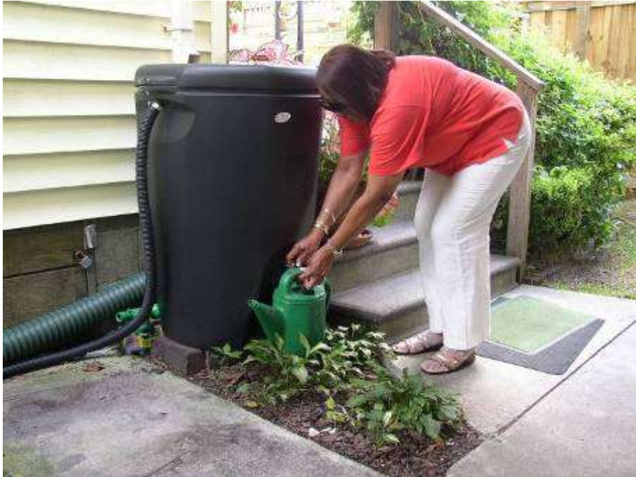
Wilmington, North Carolina Source: Tetra Tech Figure 3-25. Residential rain barrel.
