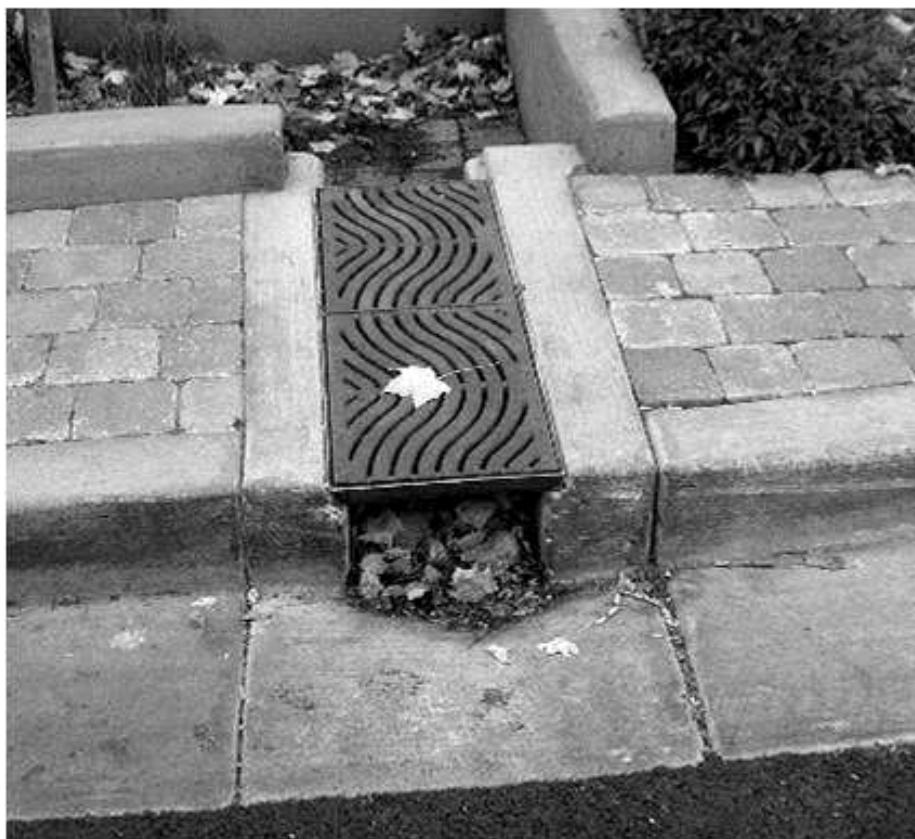
Figure 4-7. Inlet sump to remove gross solids.
