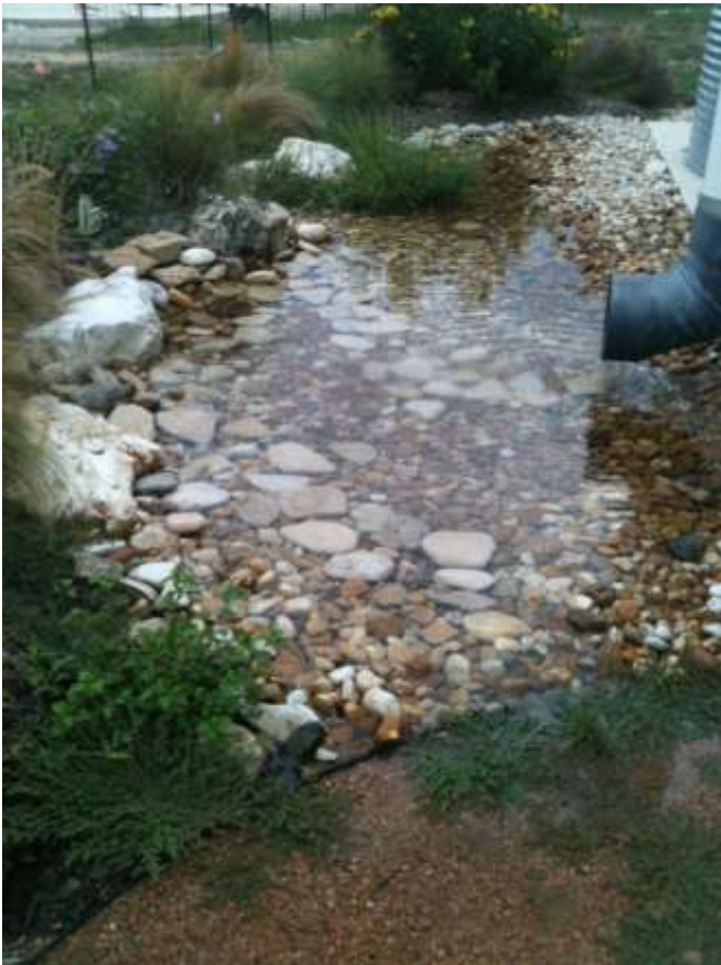
Figure B-1-16. Overflow from a rainwater cistern is discharged to a cobbled bioretention area.
