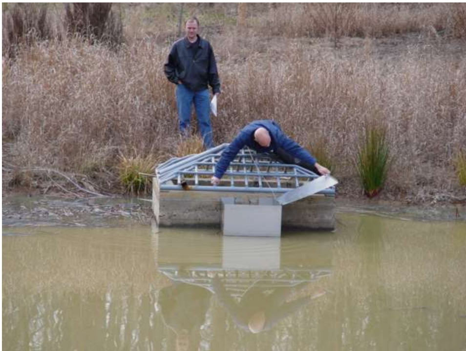
Figure B-11-16. Outlet structure with a trash rack and protected drawdown orifice.
