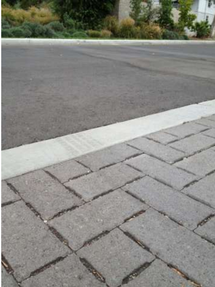
Figure B-3-14. A 1-foot concrete transition strip is used as an edge restraint between PICP and impermeable asphalt.
