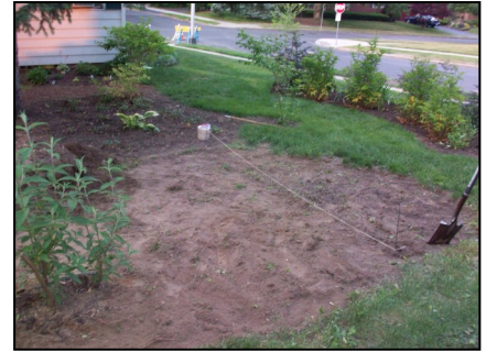
Area measured to get sense of natural slope and needed height of berm.
