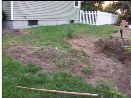
Owner of white house builds rain garden. First, garden area is scraped of grass and weeds.
