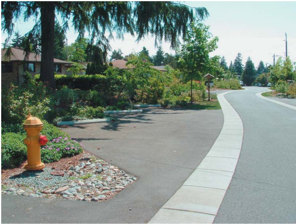
Figure 3.9 Pullout parking adjacent to a 14-foot residential access road, Seattle.
