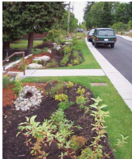
Figure 6.1.5 (left) Off-line bioretention area adjacent to roadside swale. Photo by Larry Coffman
