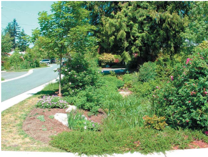
Figure 3 SEA Street bioretention swale. Photo by Colleen Owen
