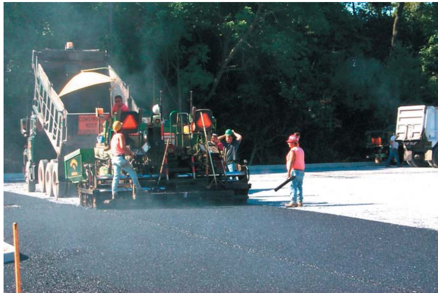
Figure 1 Parking installation, Courtesy of Cahill Associates
