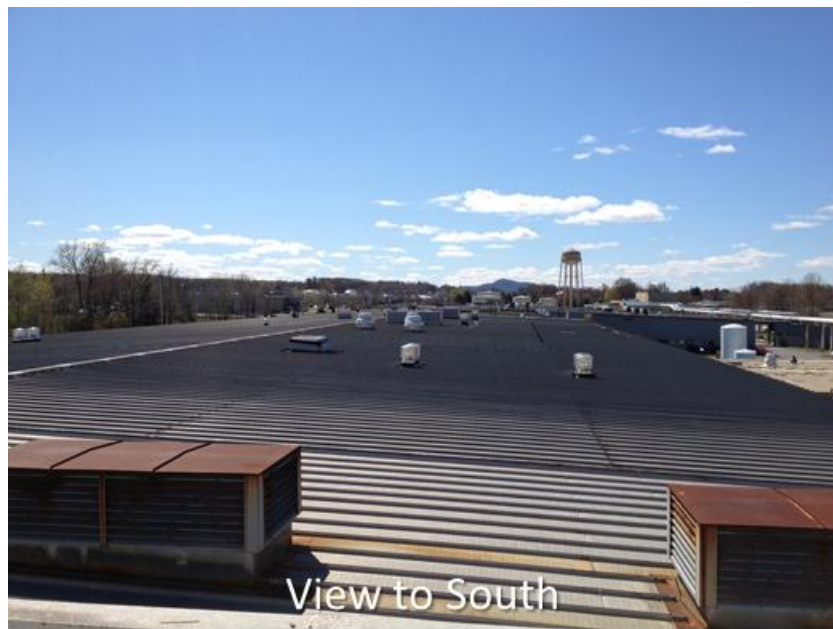
Figure 9. View of the feasible area for roof-mounted PV on Building 43 at the TechCity East Campus. Photos by James Salasovich, NREL
