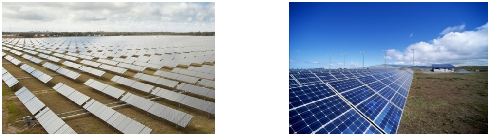
Figure 3. Mono- and multi-crystalline solar panels. Photos by (left) SunPower Corporation, NREL 23816 and (right) SunPower, NREL 13823
