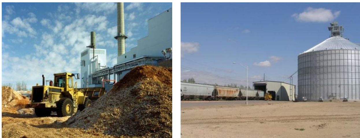
Figure 24. Biomass storage options: (left) a fuel yard and (right) a fuel silo. Photos by (left) Warren Gretz, NREL 04736 and (right) Gerry Harrow, NREL 15041
