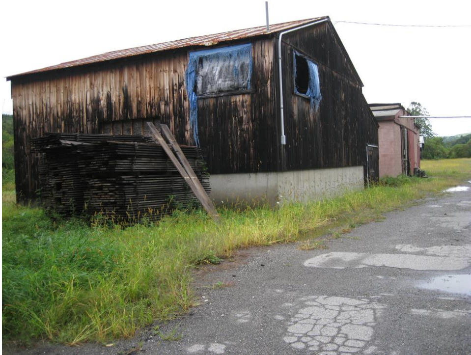
Figure 8. Two of the site buildings. Photo by Randolph Hunsberger, NREL
