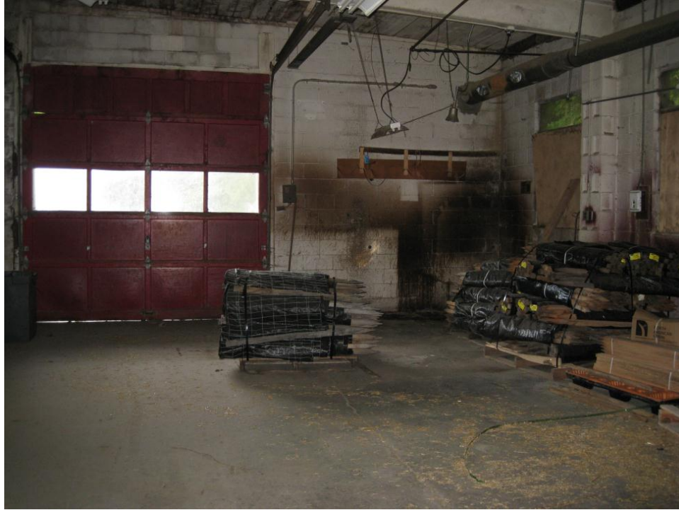
Figure 9. Inside one of the site buildings. Photo by Randolph Hunsberger, NREL
