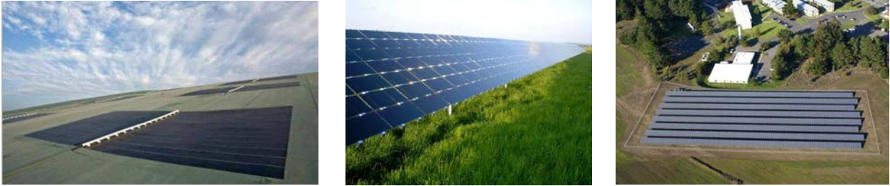
Figure 4. Thin-film solar panels installed on (left) solar energy cover and (middle and right) fixed-tilt mounting system. Pictures from (left) Republic Services, Inc., NREL 23817; (middle) Beck Energy, NREL 14726; and (right) U.S. Coast Guard Petaluma site, NREL 17395
