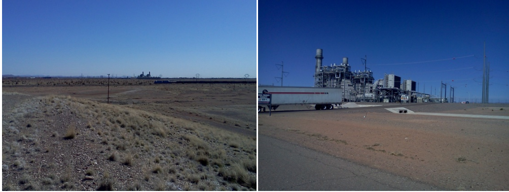
Figure 9. Electrical tie-in point for the PV system at the 345-kV line or the substation. Photos by Kosol Kiatreungwattana, NREL
