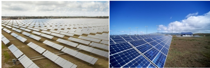
Figure 3. Mono- and multi-crystalline solar panels. Photos from (left) SunPower Corporation, NREL 23816 and (right) SunPower, NREL 13823
