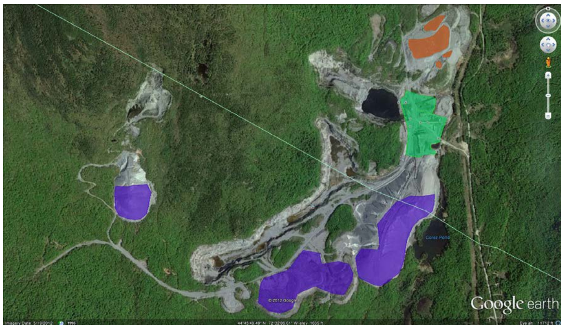
Figure 9. Aerial view of the feasible area for PV at the VAG Mine site
