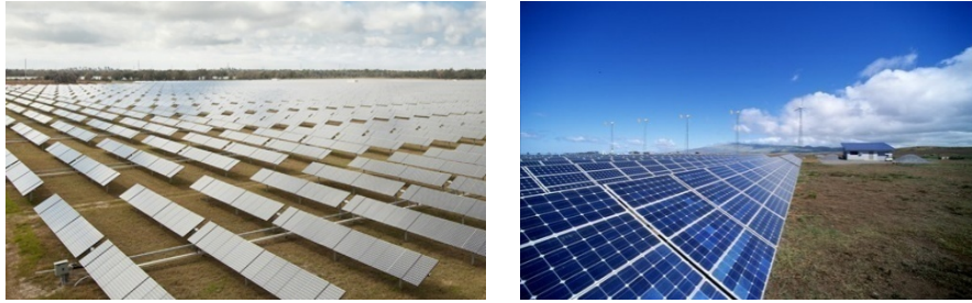
Figure 5. Mono- and multi-crystalline solar panels. Photos from (left) SunPower Corporation, NREL 23816 and (right) SunPower, NREL 13823
