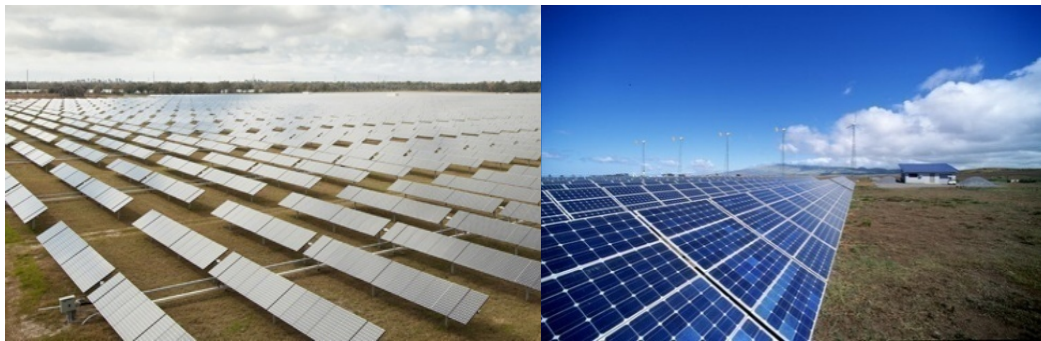
Figure 3. Mono- and multi-crystalline solar panels. Photos by (left) SunPower Corporation, NREL 23816 and (right) SunPower, NREL 13823
