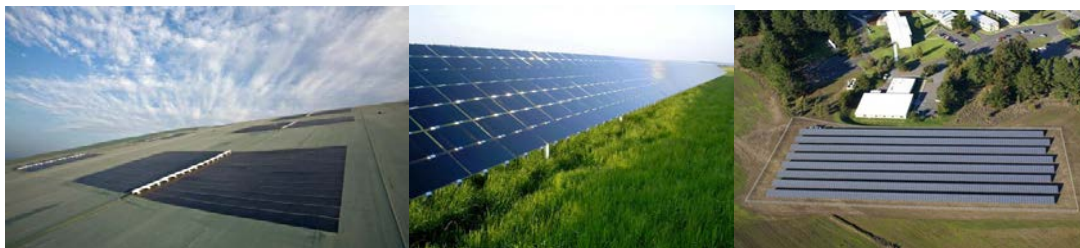
Figure 4. Thin-film solar panels installed on (left) solar energy cover and (middle/right) fixed-tilt mounting system. Photos by (left) Republic Services, Inc., NREL 23817, (middle) Beck Energy, NREL 14726, and (right) U.S. Coast Guard Petaluma Site, NREL 17395
