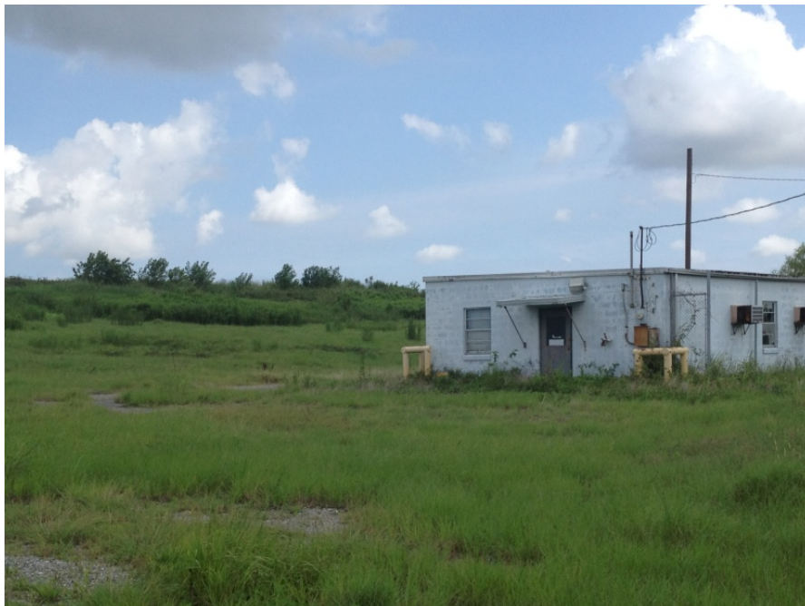
Figure 3. Photo of the south side of the site. Photo by Kristi Moriarty, NREL
