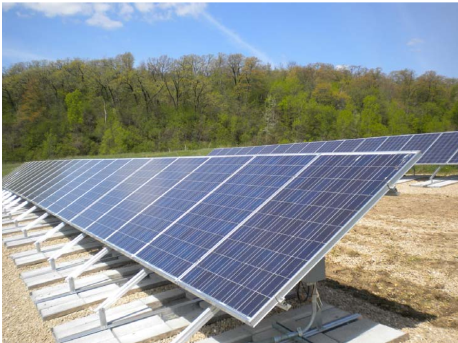
Figure 5. View of the 10 kW ballasted PV system currently at the Refuse Hideaway Landfill
