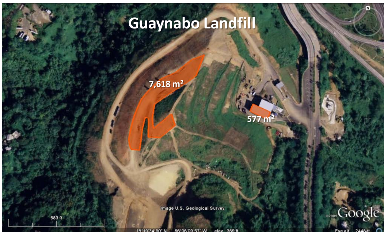
Figure 14. Aerial view of the feasible area for PV at the Guaynabo Landfill and recycling center
