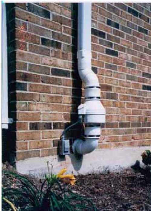
Figure IV-3: Fan/blower and discharge piping
