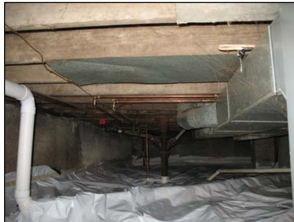
Piping in crawl space
