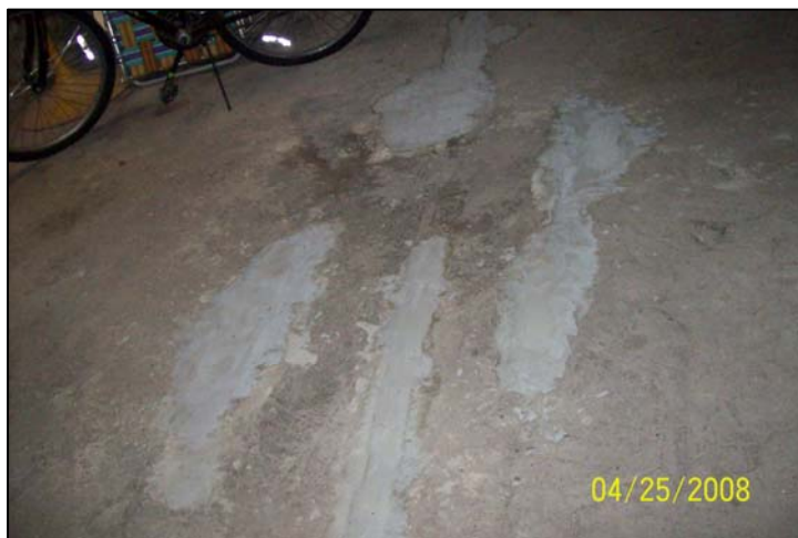
Sealed cracks in basement floor
