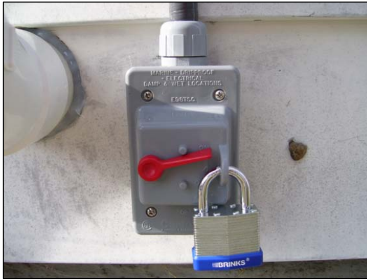
Deadbolt that locks the SSDS switch in the “on” position
