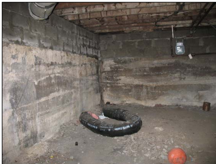
Basement with dirt floor
