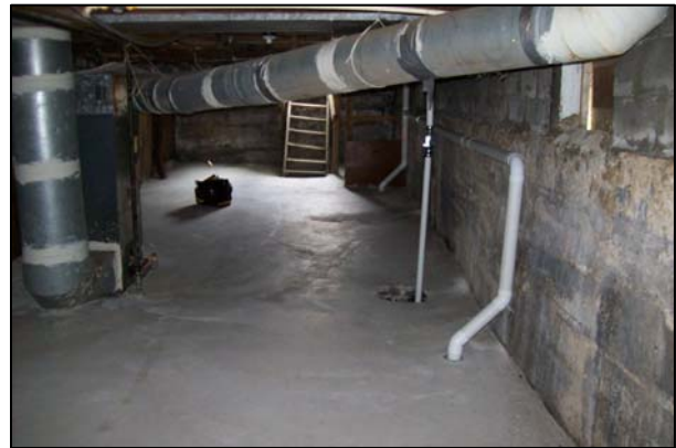
Basement with new concrete floor and SSDS
