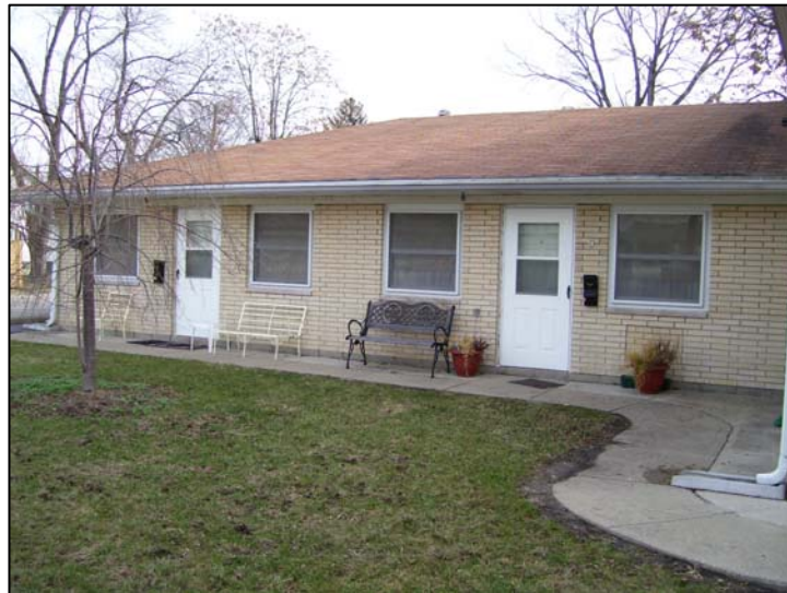
Property on slab foundation with no basement
