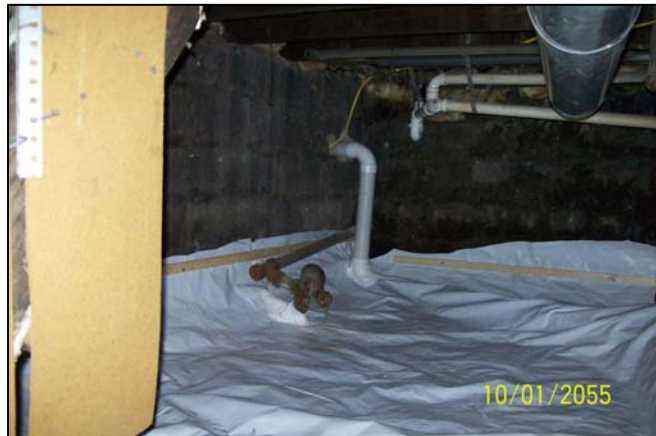
Piping beneath membrane
