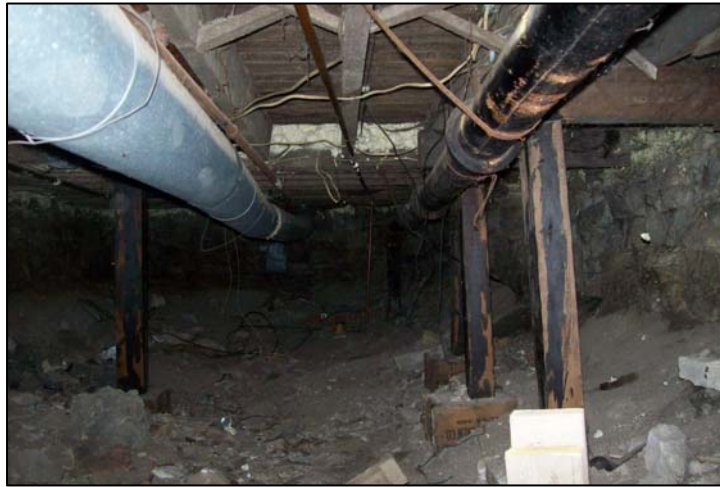
Dirt crawl space beneath foundation
