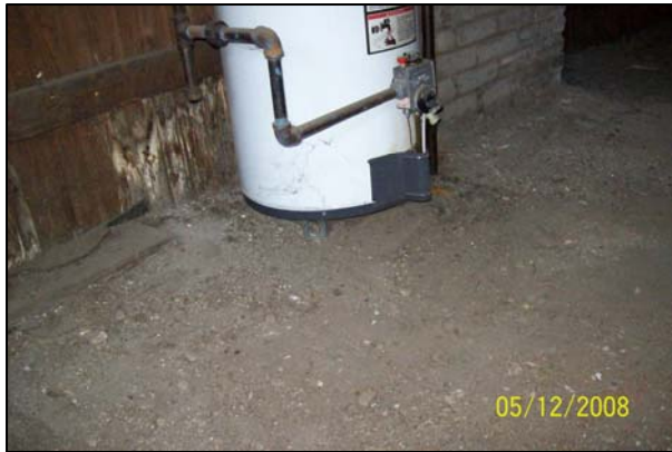
Basement with dirt floor
