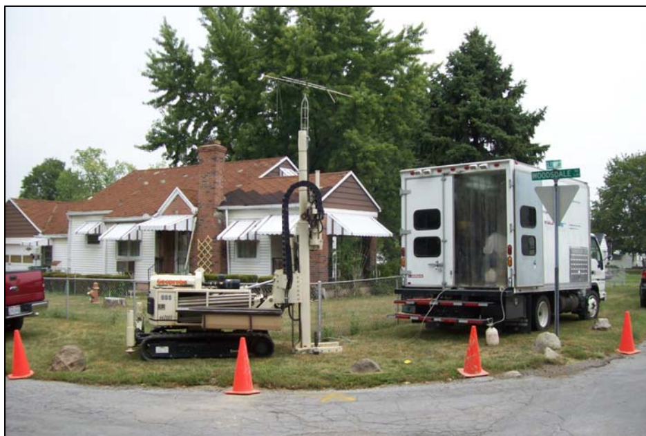
First Step - Geoprobe obtaining a groundwater sample
