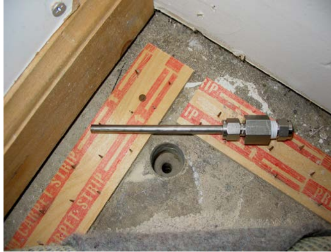
Assembled subslab port ready for installation
