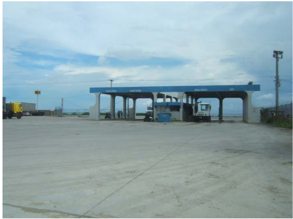
Photo description: yard entrance gate and control point
