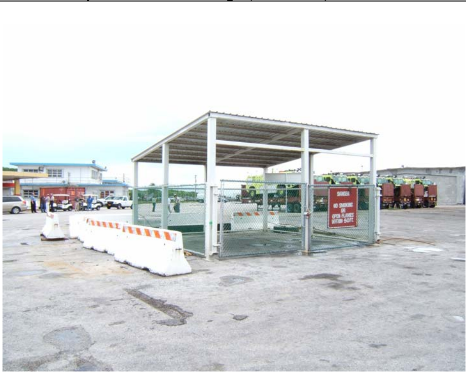
Photo description: Hazard storage (behind W2)
