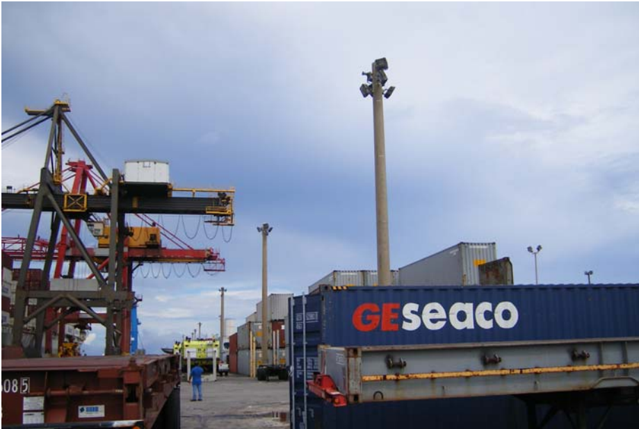
Photo description: Pole mounted yard lighting
