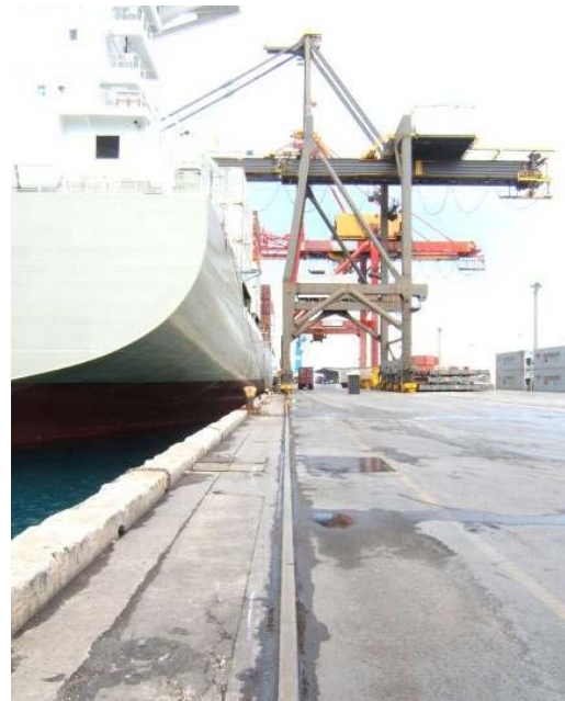
Crane Rails at F-4, F-5 and F-6
