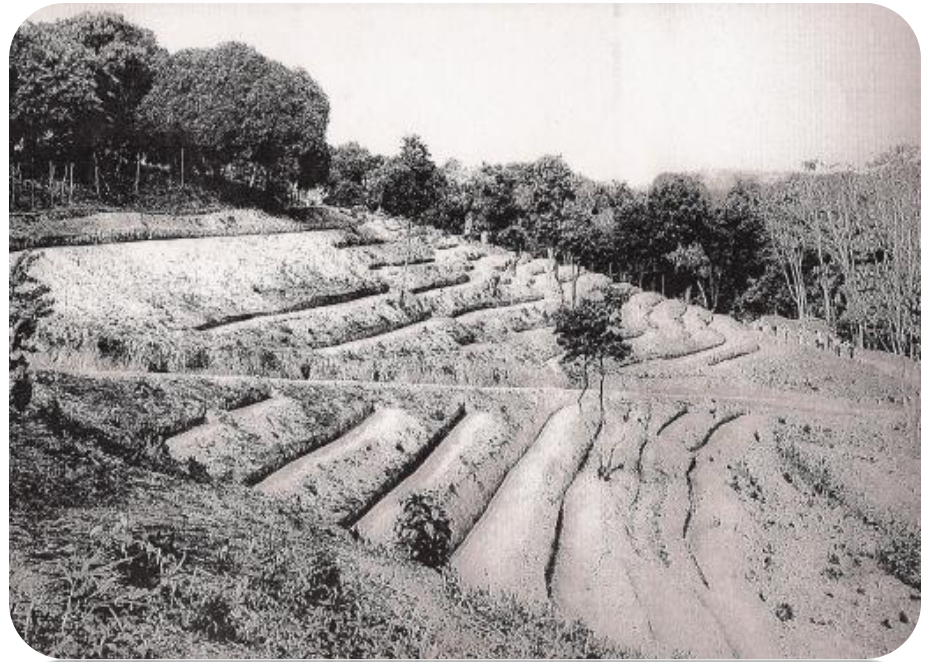
Contour bench terraces at the Soil Erosion Station, Mayagüez. "Las Ochenta Farm". 1936-38
