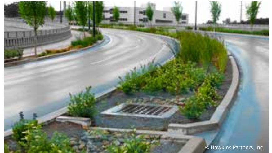
In Nashville, Tennessee the combined city and county government has experimented with green streets in three locations, all with positive public response. This is 28th/31st Avenue Connector which was completed in 2012. The blue shows where the water runs during storms.
