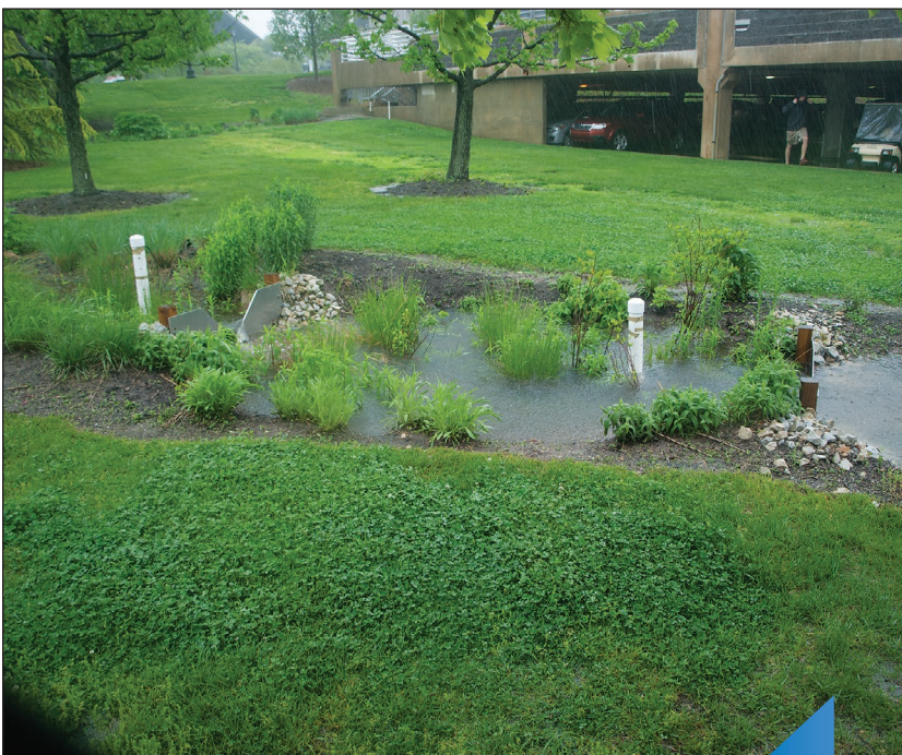
Bioretention rain garden at Villanova, Pennsylvania. Since 1999, the Villanova Urban Stormwater Partnership has constructed and monitored multiple innovative BMP devices, including a stormwater wetland, bioinfiltration and bioretention rain gardens, pervious concrete/porous asphalt installations, an infiltration trench, a treatment train and a green roof.
