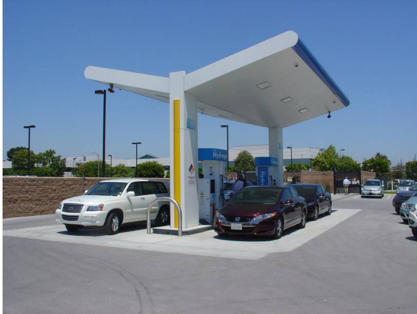
Figure 3.6.4 Fueling station using pipeline hydrogen - If a hydrogen pipeline is located nearby, the cost of building the hydrogen production system can be avoided, lowering the cost of dispensed hydrogen (photo source: NREL).
