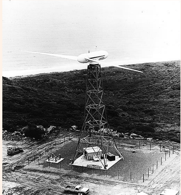
A wind turbine generator being field tested on Culebra Island, Puerto Rico for the Department of Energy and NASA. Photo circa 1978.
