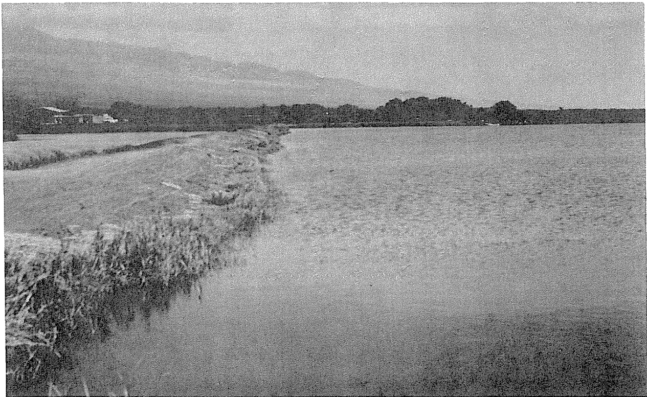
Figure 4. 'Tropic Shore' stabilizing an aquaculture pond bank at the Maui County Agricultural Research Park, Kihei, Maui. Stolons were planted at or slightly below the water level. This planting is three months old.
