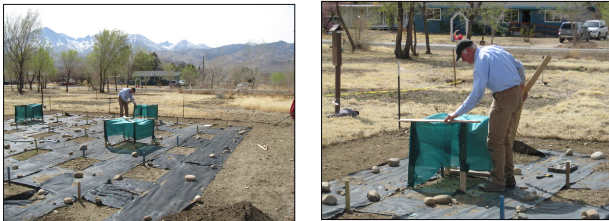
Figure 8. Installation of shade fabric structures for selected plots at the BPPT Nahavita Conservation Field Trial, March 2013, Big Pine, CA.
